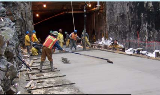
Laying Concrete Invert
