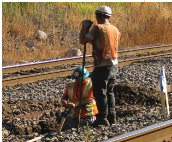
Hand Digging for Catenary Foundation.
