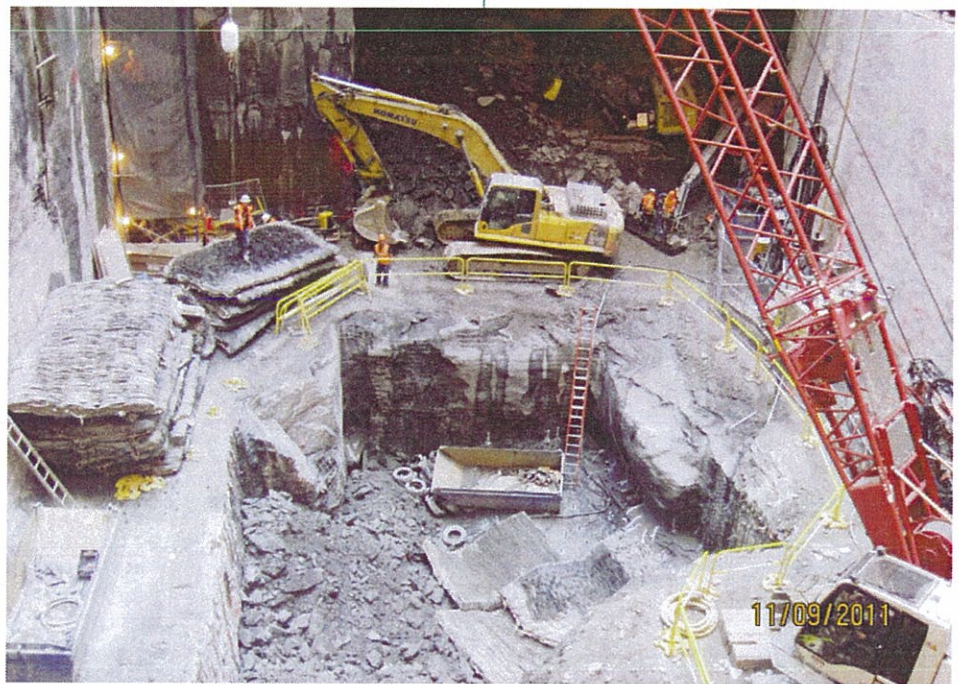
Preparing for Next Blast in the Shaft
