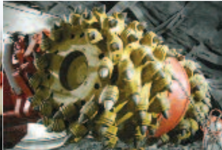
Road header excavation of cavern
