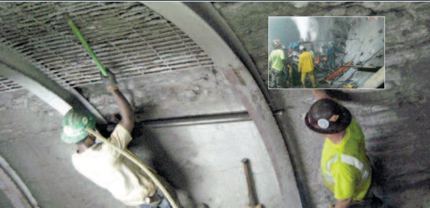
Shooting shotcrete to support tunnel section
