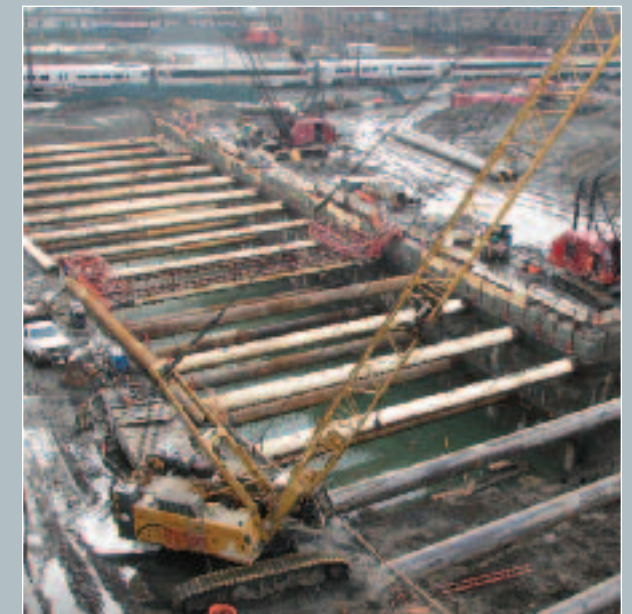
Open-cut excavation in Queens
