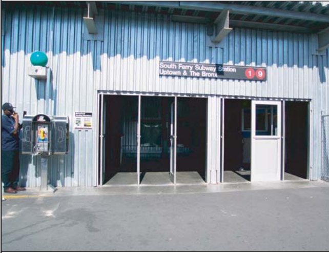
South Ferry Station exterior.
