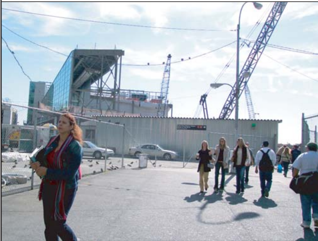
South Ferry Station with Whitehall Ferry Terminal reconstruction in background.
