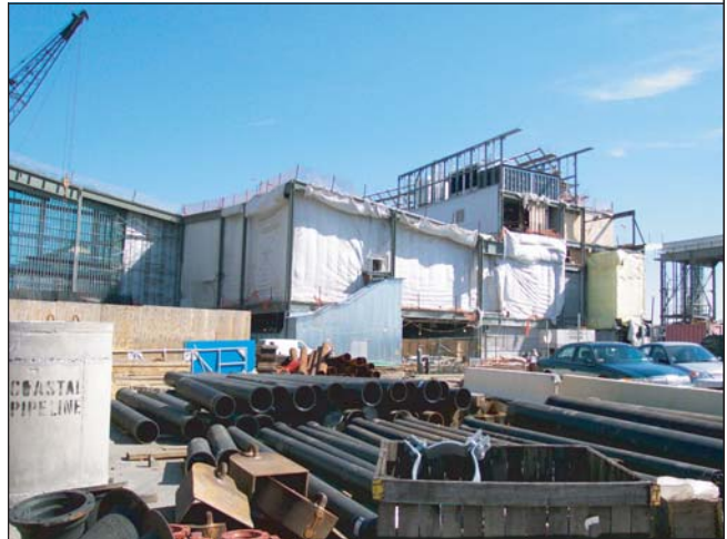
Whitehall Ferry Terminal reconstruction.
