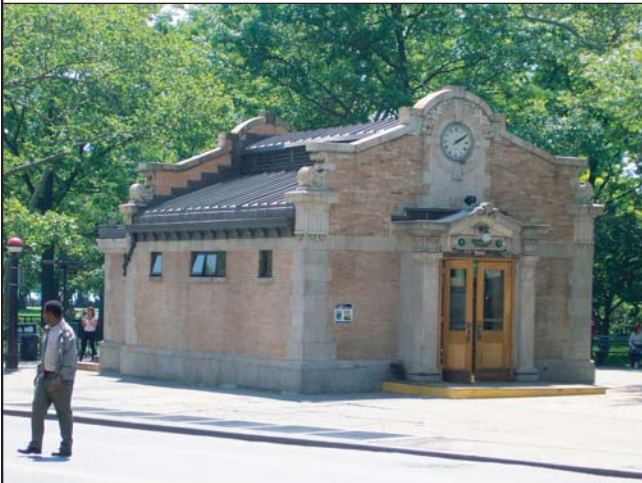
IRT Bowling Green Control House, looking southwest to Battery Park from State Street.
