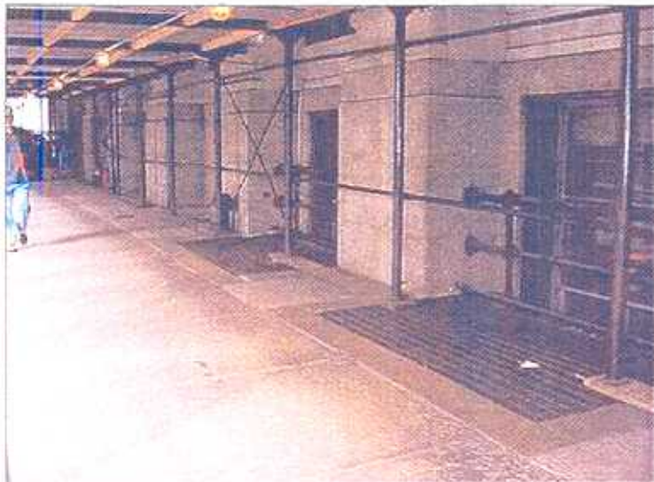
PHOTO 4- GREENWICH STREET SIDEWALK AND WINDOW WELLS
