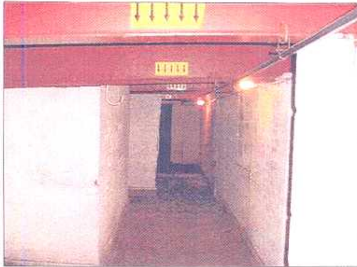
PHOTO 5- INSIDE VAULT, FACING NORTH UNDER GREENWICH STREET SIDWALK
