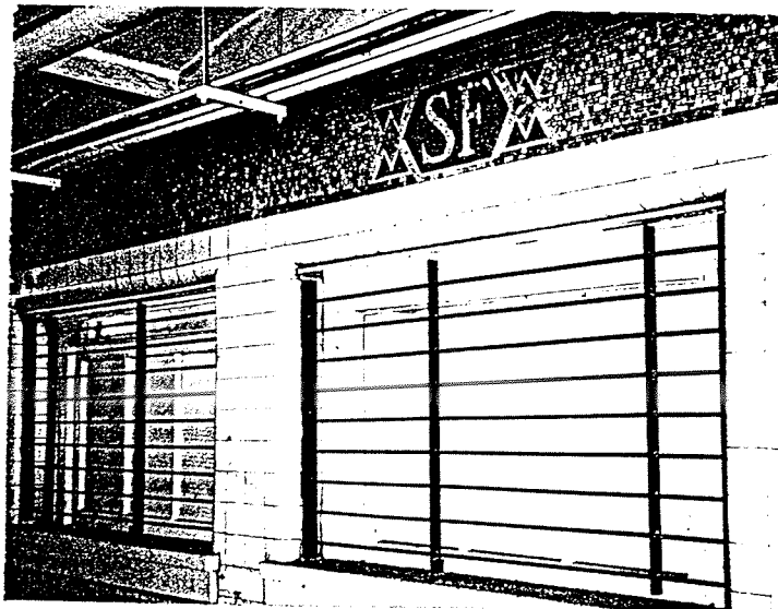
South Ferry Station: Platform Walls on 1918 Inner Loop Showing Original Mosaic Banding.
