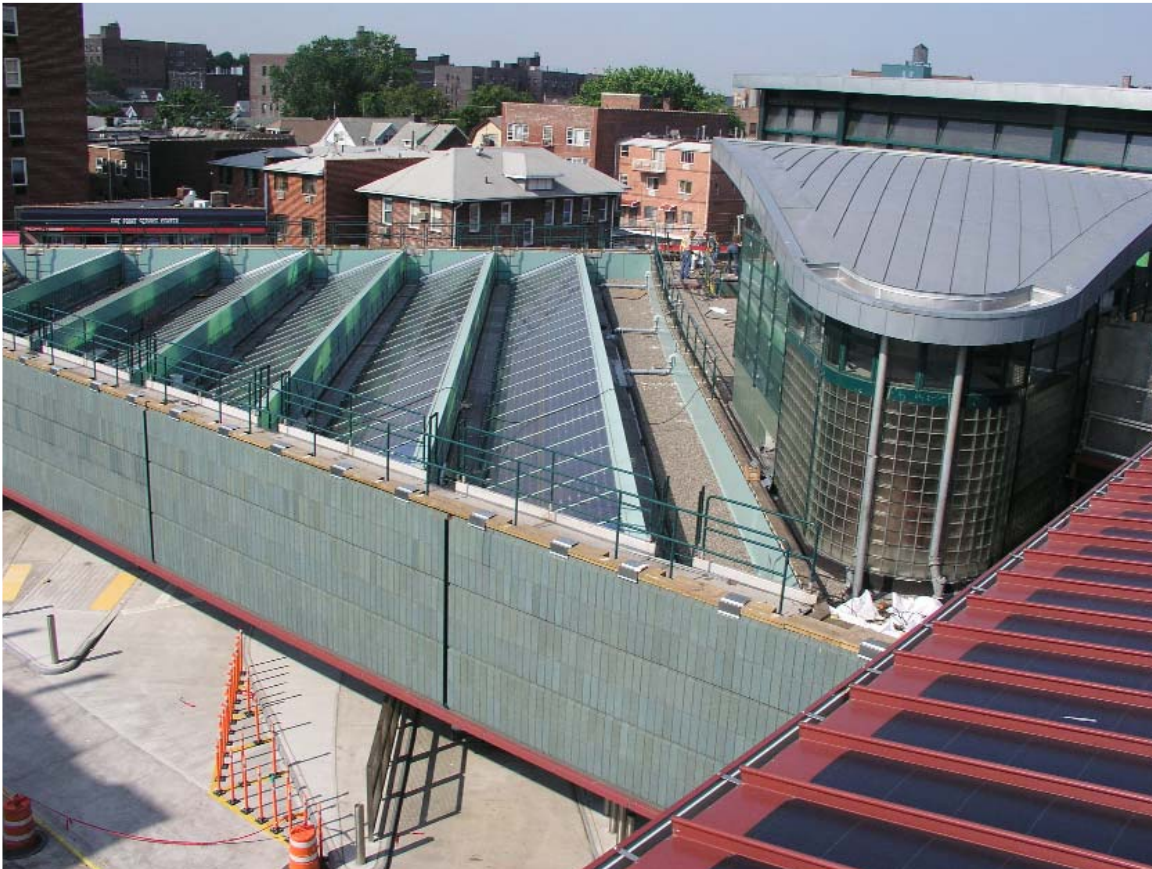
Solar Roof, Roosevelt Avenue Station, MTA New York City Transit
