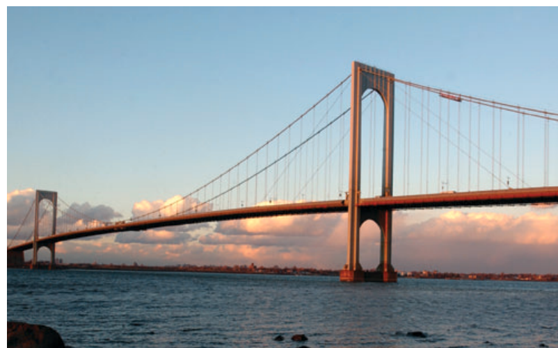
The restored 1939 profile of the Bronx-Whitestone Bridge.
