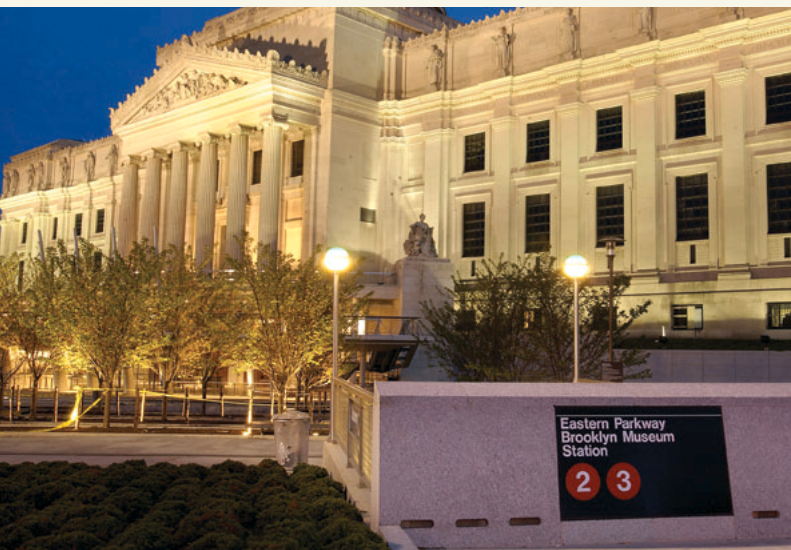
The new subway entrance at the Brooklyn Museum.
