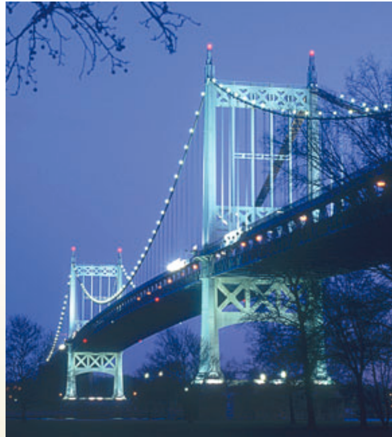
A steel deck replaced the concrete roadway on The Triborough Bridge in 2004.
