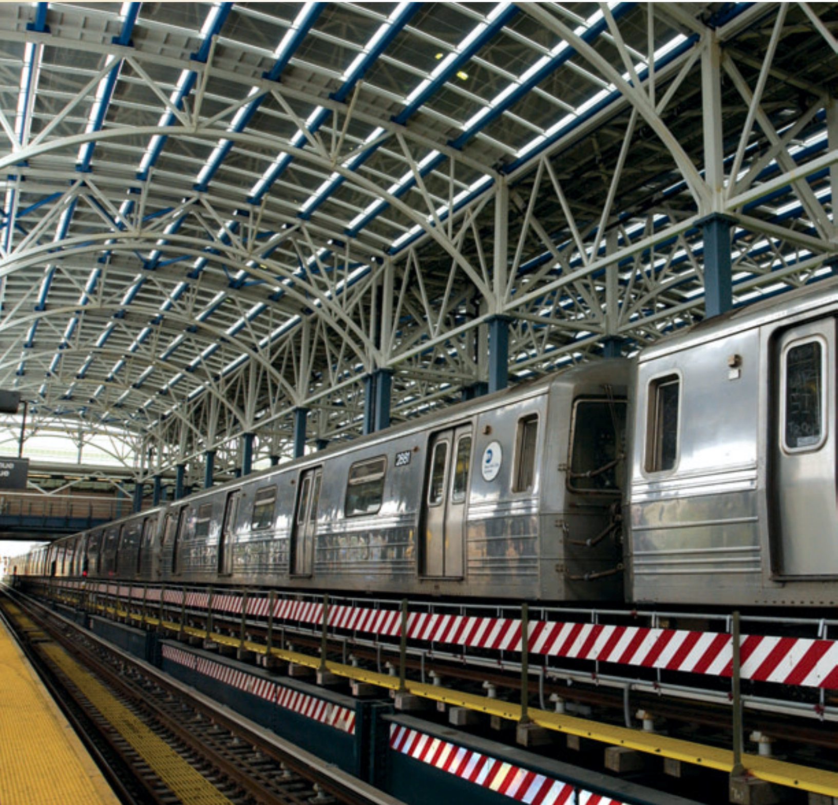
The rehabilitated Stillwell Avenue terminal at Coney Island.
