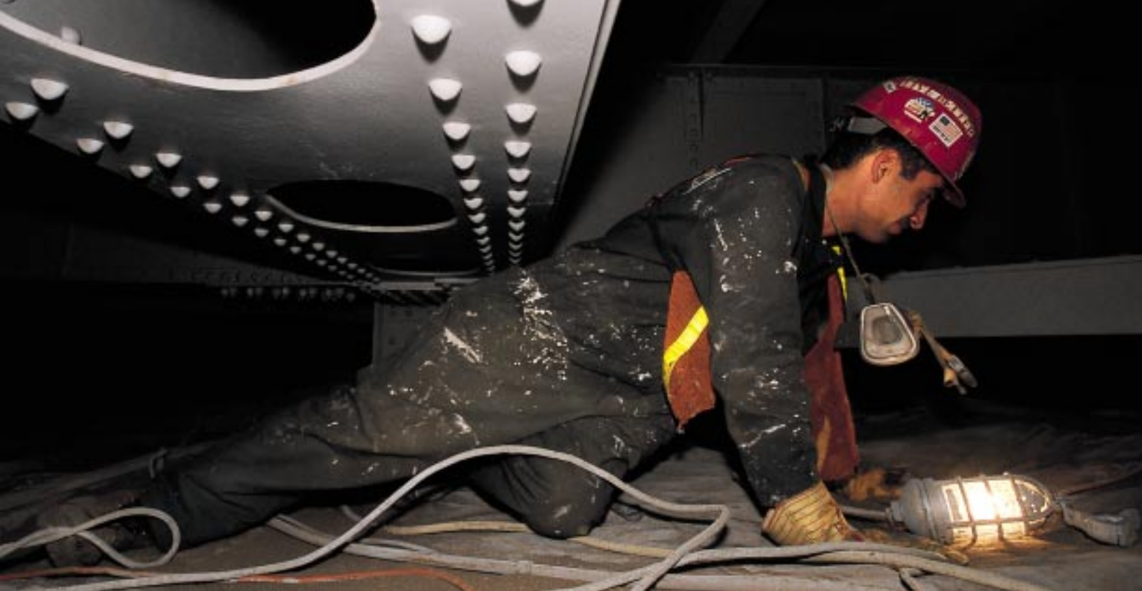
Putting the finishing touches on repainting of the Verrazano-Narrows Bridge
