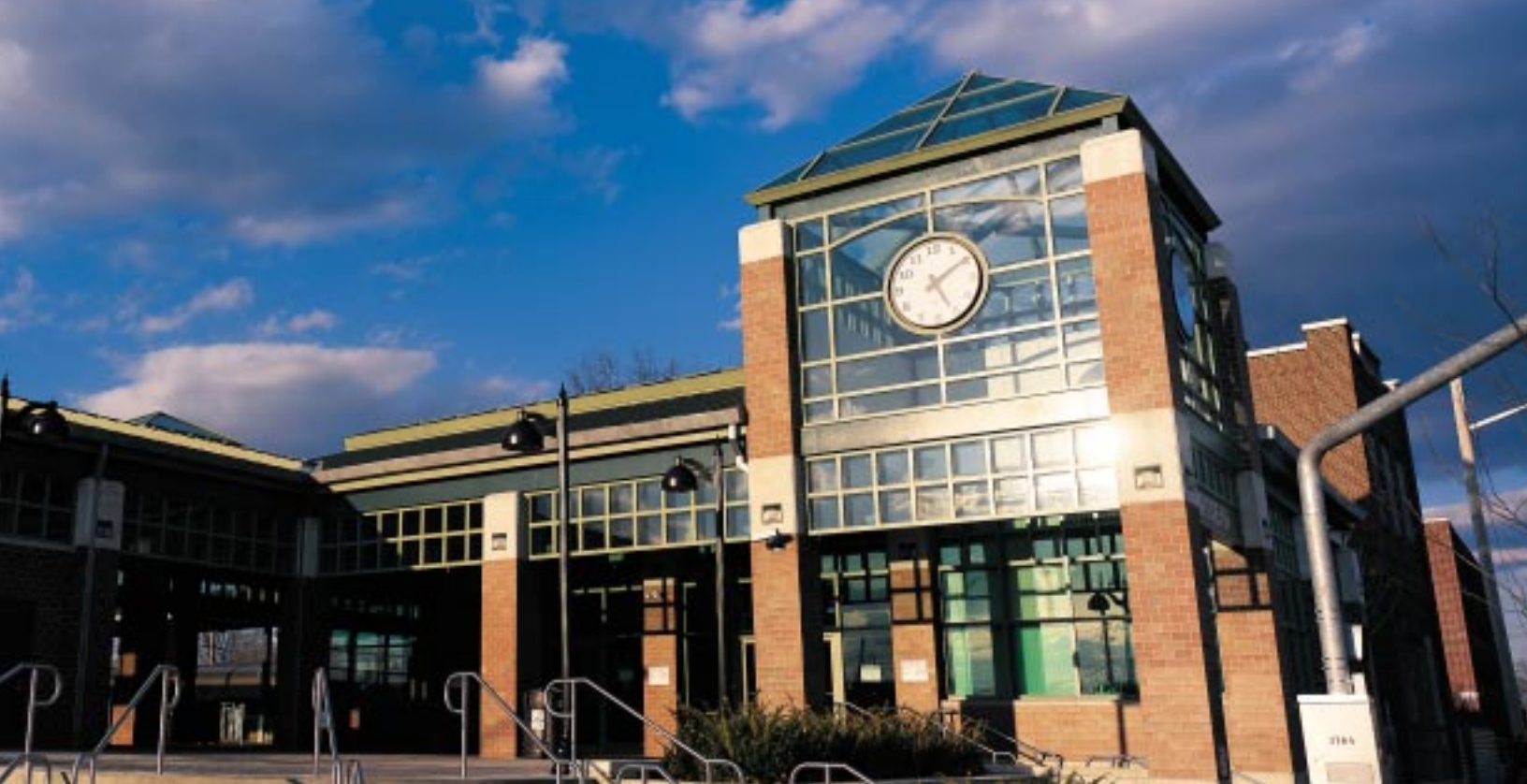
The new LIRR Hempstead Station
