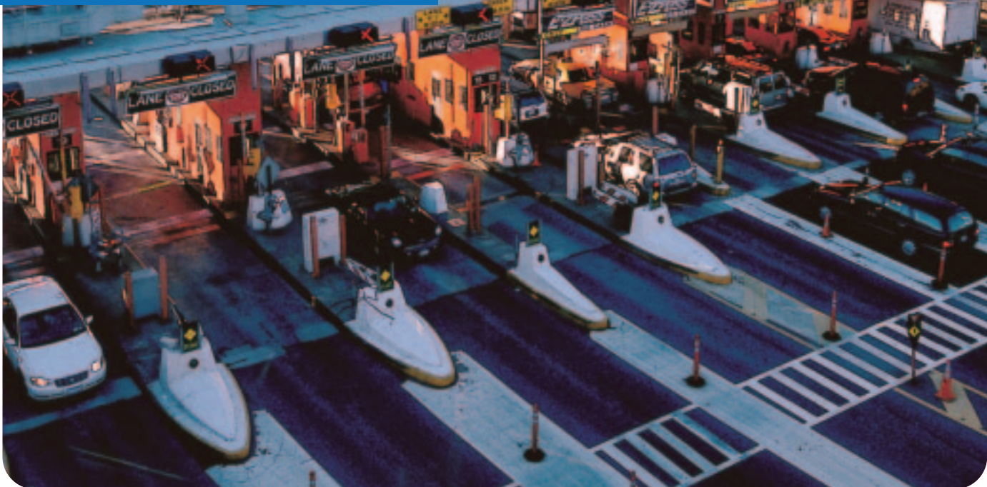
Queens Midtown Tunnel Toll Plaza
