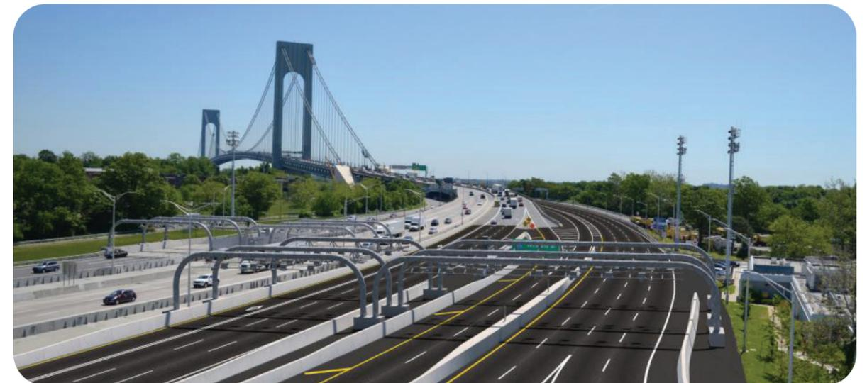
Figure 25 Toll gantries (the arched metal structures over the roadways) at the Verrazzano-Narrows Bridge
