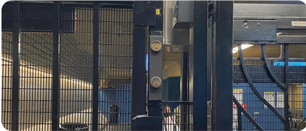
Figure 24 At Jamaica Center-Parsons Archer station, typical emergency exit gate locks as seen from the unpaid side. All these locks are in the process of being replaced across the subway system because excessive unauthorized duplication of keys has made the locks a pathway to fare evasion.
