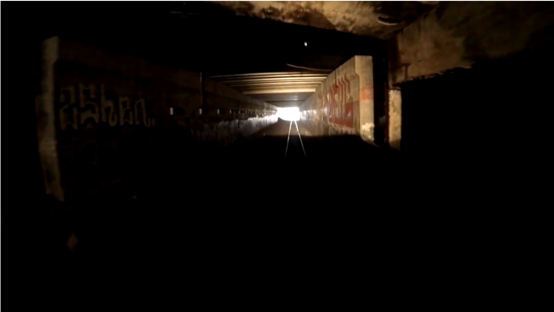
BIN: N/A Name: Overbuild b/w Flatbush and Nostrand Avenues
