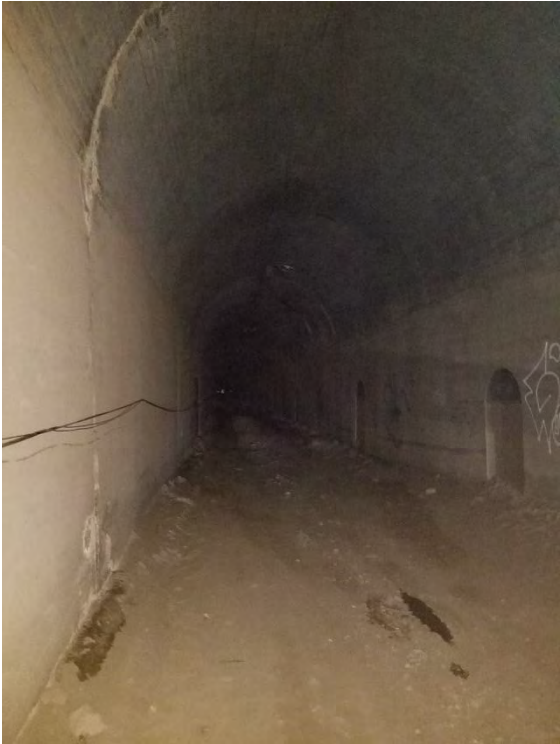
Picture 10 – Inside out-of-service tunnel on west side
