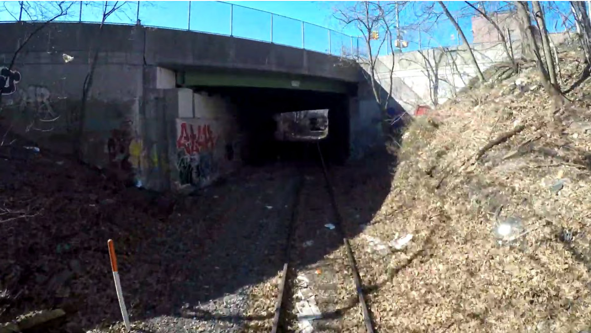
BIN: 2243360 Name: 17. 16 th Avenue/59 th Street
