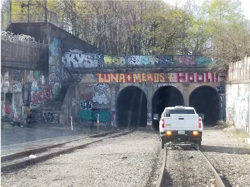
Picture 1 – View of East New York Tunnel entry, looking south
