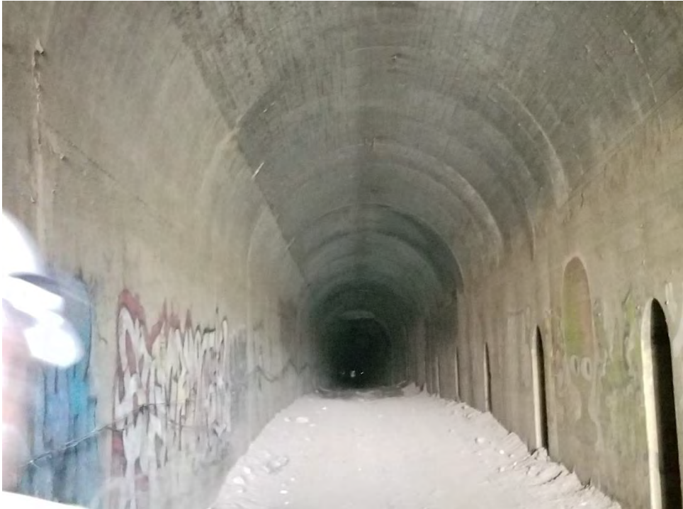
Picture 5 – Out-of-service tunnel depicting openings to adjoining tunnel
