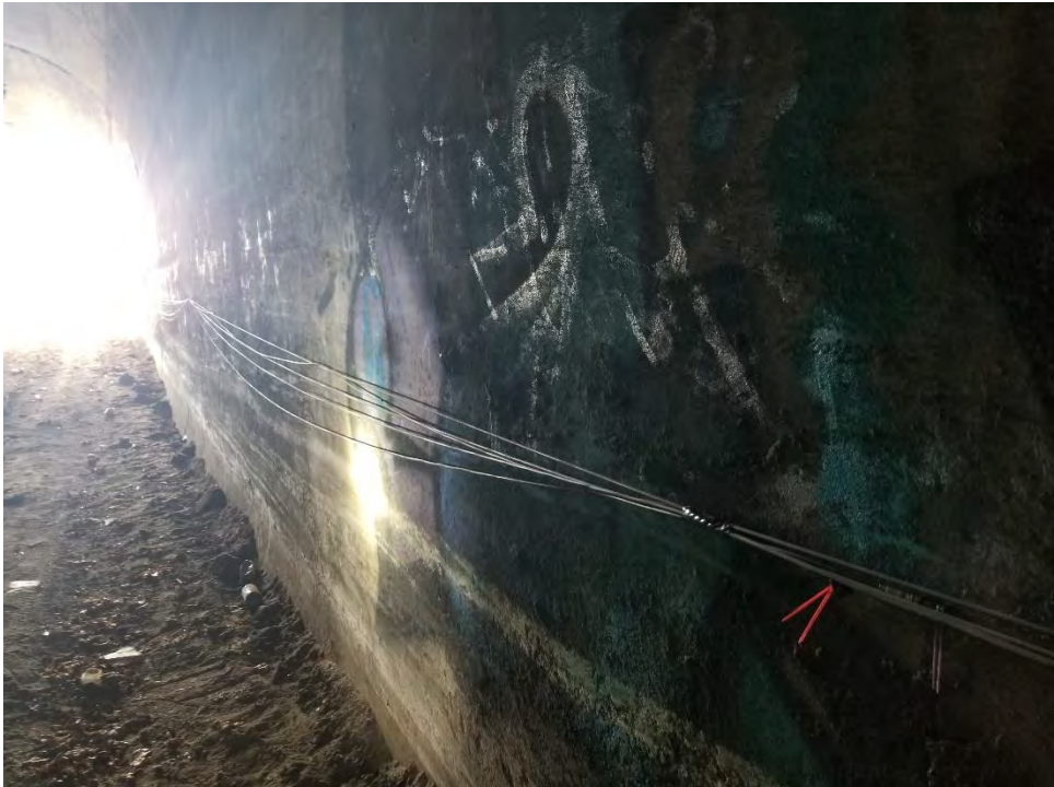
Picture 6 – Inactive tunnel, looking south
