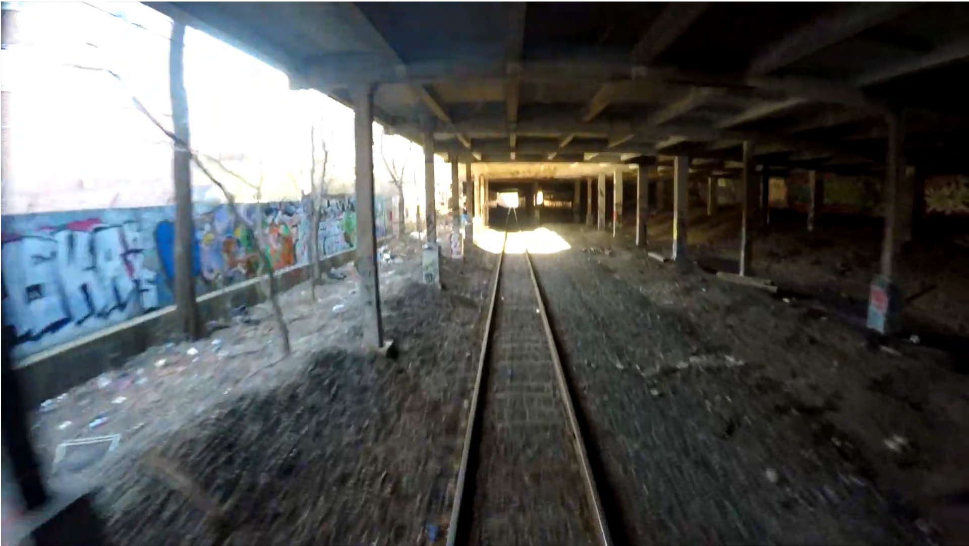
BIN: N/A Name: Parking Overbuild East of Flatbush Avenue
