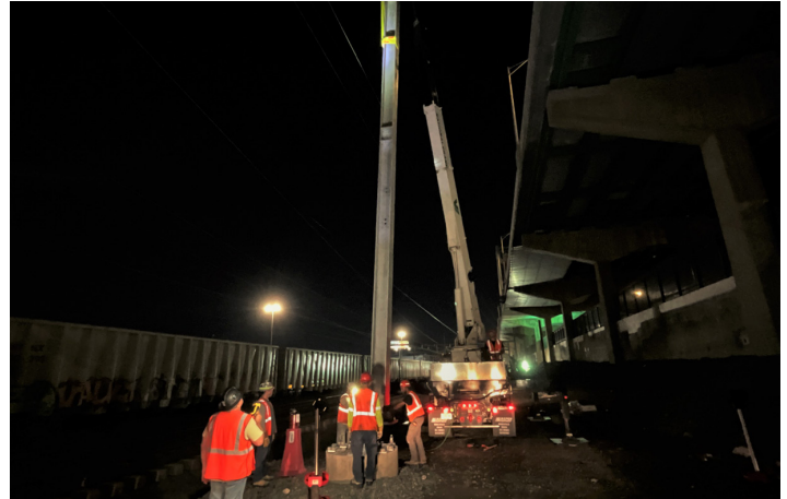
PSA construction workers erect OCS column portal, July, 2023
