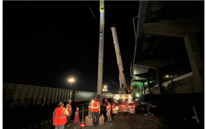
*PSA construction workers erect OCS column portal
