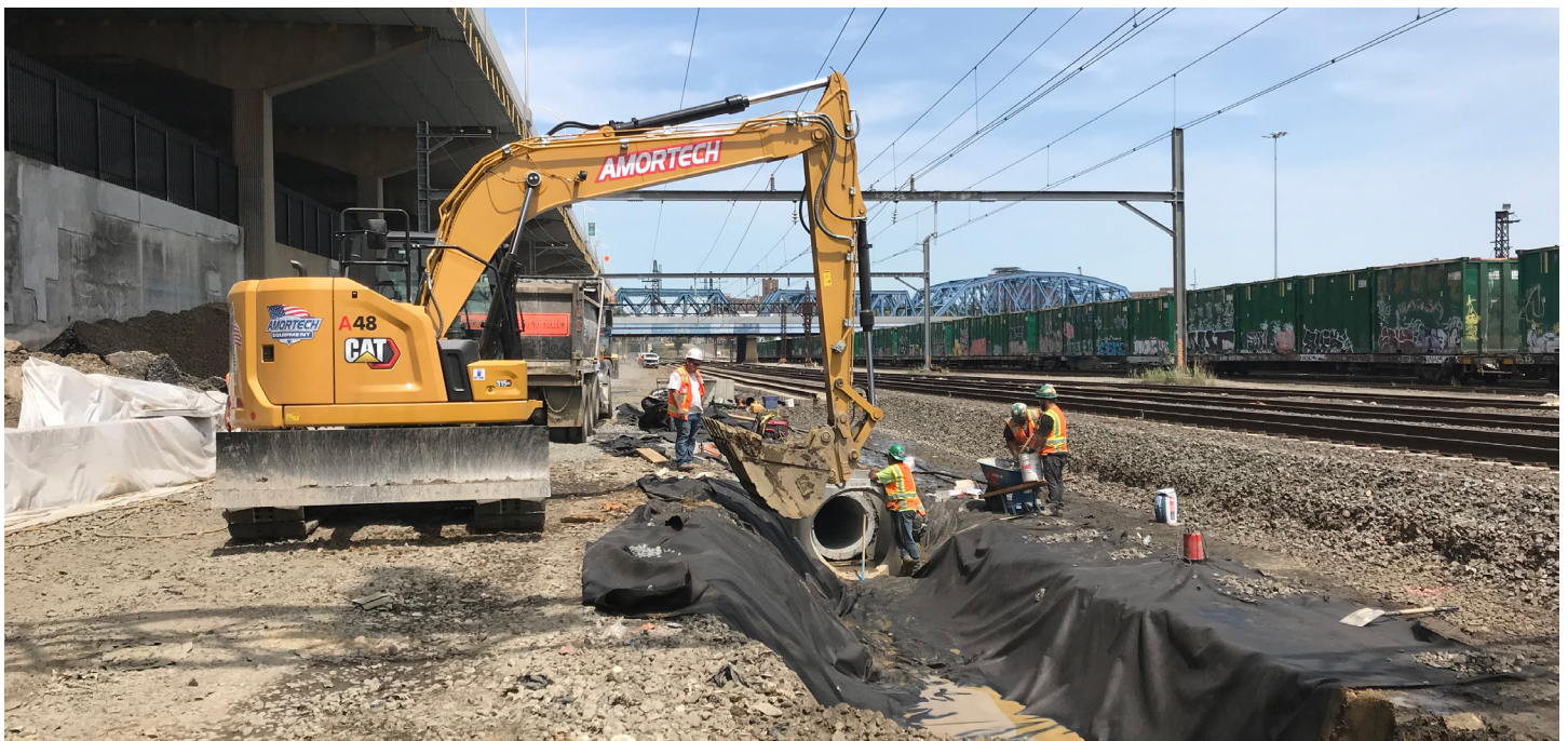
PSA construction workers install drainage system near Leggett Interlocking, May, 2023
