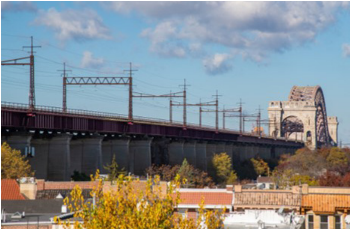
The existing OCS structures along the project corridor, November, 2022
