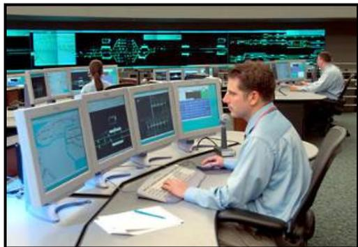
These next 20 years will see much of the subway signal system rebuilt with communications-based train control (CBTC), an advanced signal system that enables real-time centralized train supervision and monitoring, permitting trains to operate with shorter headways, thus increasing capacity. It also provides for automated train operation and information regarding the
