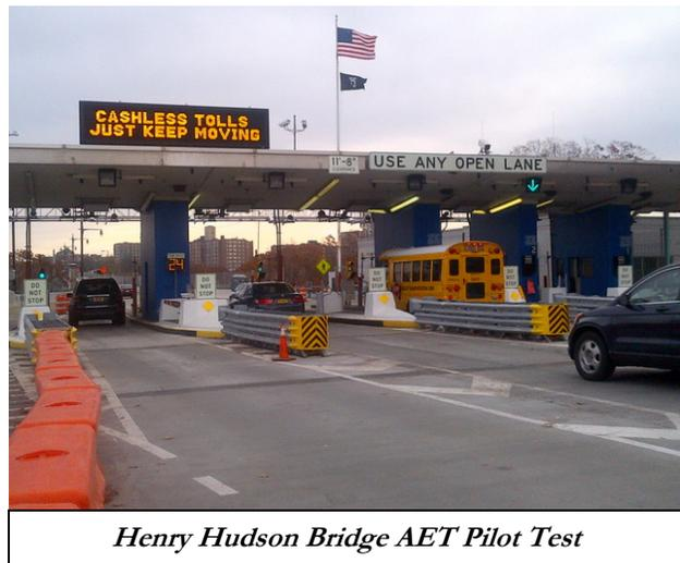
purpose of the pilot is to test both the new technologies required to collect video images from passing vehicles and the back-office systems to collect tolls from registered owners of vehicles without an E-ZPass tag. The pilot will also help determine the operational and financial issues in a cashless environment. The data collected from this pilot will be used to evaluate and guide future toll collection and toll plaza reconstruction plans.
