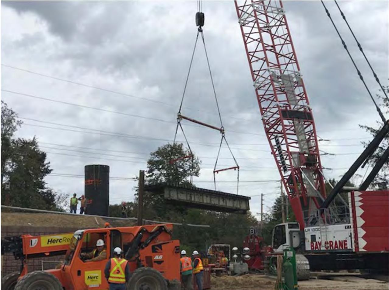
**Accabonac Road Bridge Replacement:** An alternative service plan went into effect in October to support the replacement of two (2) LIRR Bridges over North Main Street and Accabonac Road in East Hampton. The replacement bridges will increase the elevation of the tracks to lower the chance of bridge strikes in the future. Service restoration is planned for November 10, 2019.
