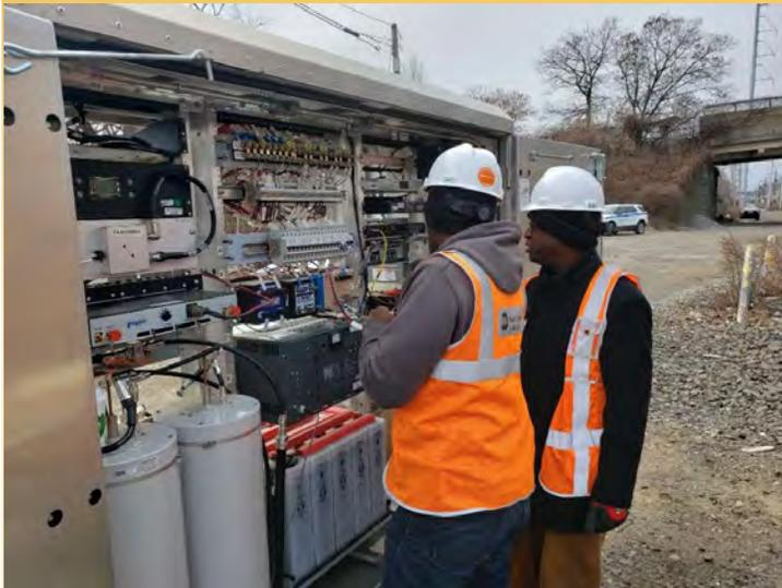
Transponder testing with Portable Testing Equipment (PTE)
