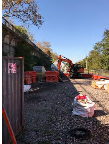
Photo 6: Contractor yard on the Proposed Alignment of Section 1 in subsection 1C, facing west (REC ID S001), and view of the eastern-most portion of the bike path.
