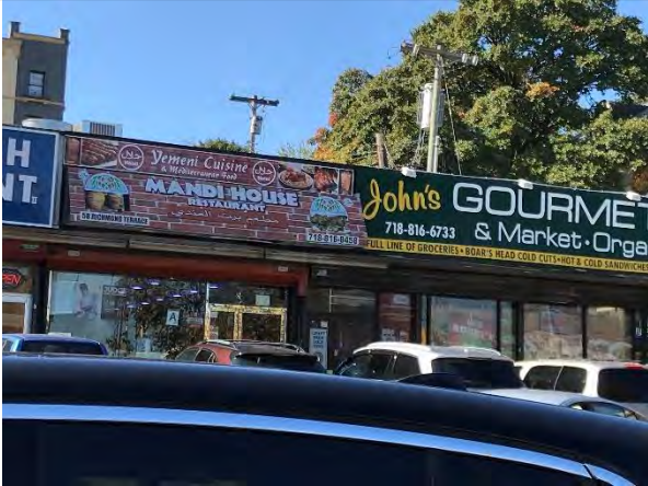
Photo 13: Commercial strip mall, located northwest-adjacent to the Proposed Alignment of Section 1, facing south.
