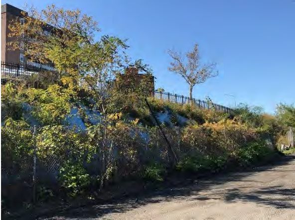
Photo 9: Piles of stockpiled soil were observed on the western portion of the Proposed Alignment of Section 1 along the Richmond Terrace retaining wall, facing southwest.
