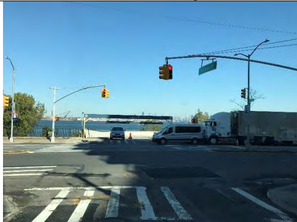
Photo 3: Richmond Terrace and Nicholas Street intersection/entrance to the northeast-adjacent St. George Terminal, facing east.
