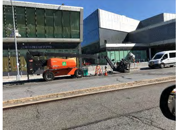
Photo 14: Construction machinery, located northeast-adjacent to the Proposed Alignment of Section 1, facing northeast.
