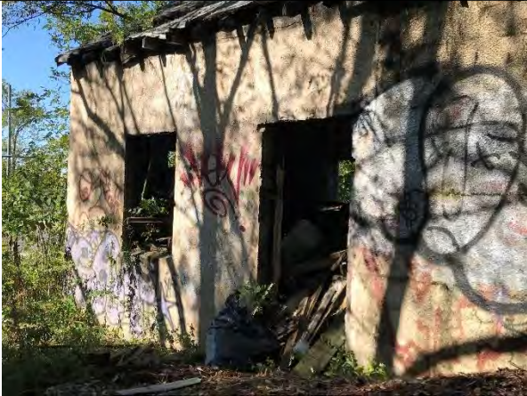
Photo 11: Potential dumping located north-adjacent to the western portion of the Proposed Alignment of Section 1, facing northwest.
