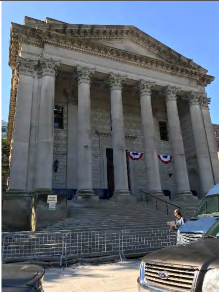
Photo 15: Staten Island Municipal Building, located southwest-adjacent to the Proposed Alignment of Section 1, facing southwest.
