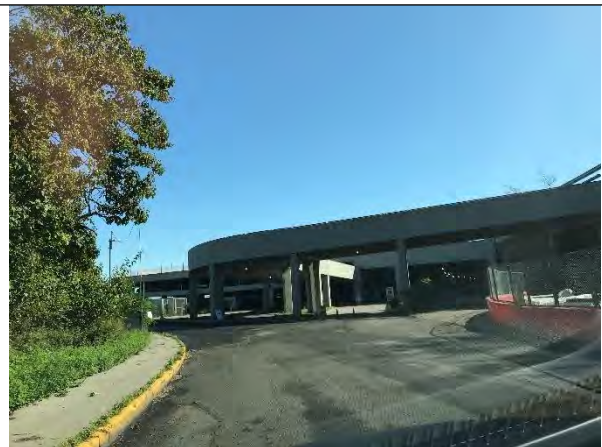
Photo 8: Access ramp to east-adjacent multilevel parking garage at the intersection of Richmond Terrace and Nicholas Street in subsection 1C, facing east.
