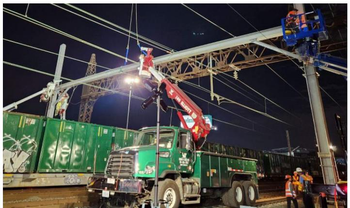
Above: PSA construction workers install OCS portal at Leggett Interlocking, October 2023
