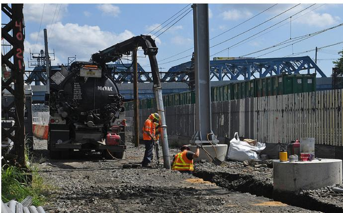
Above: Workers excavate trench for OCS cables at Leggett Interlocking, August 2023
