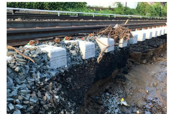
Washout from torrential rainfall flooding near Bayside on the Port Washington Branch from Tropical Storm Ida, September 2023.
