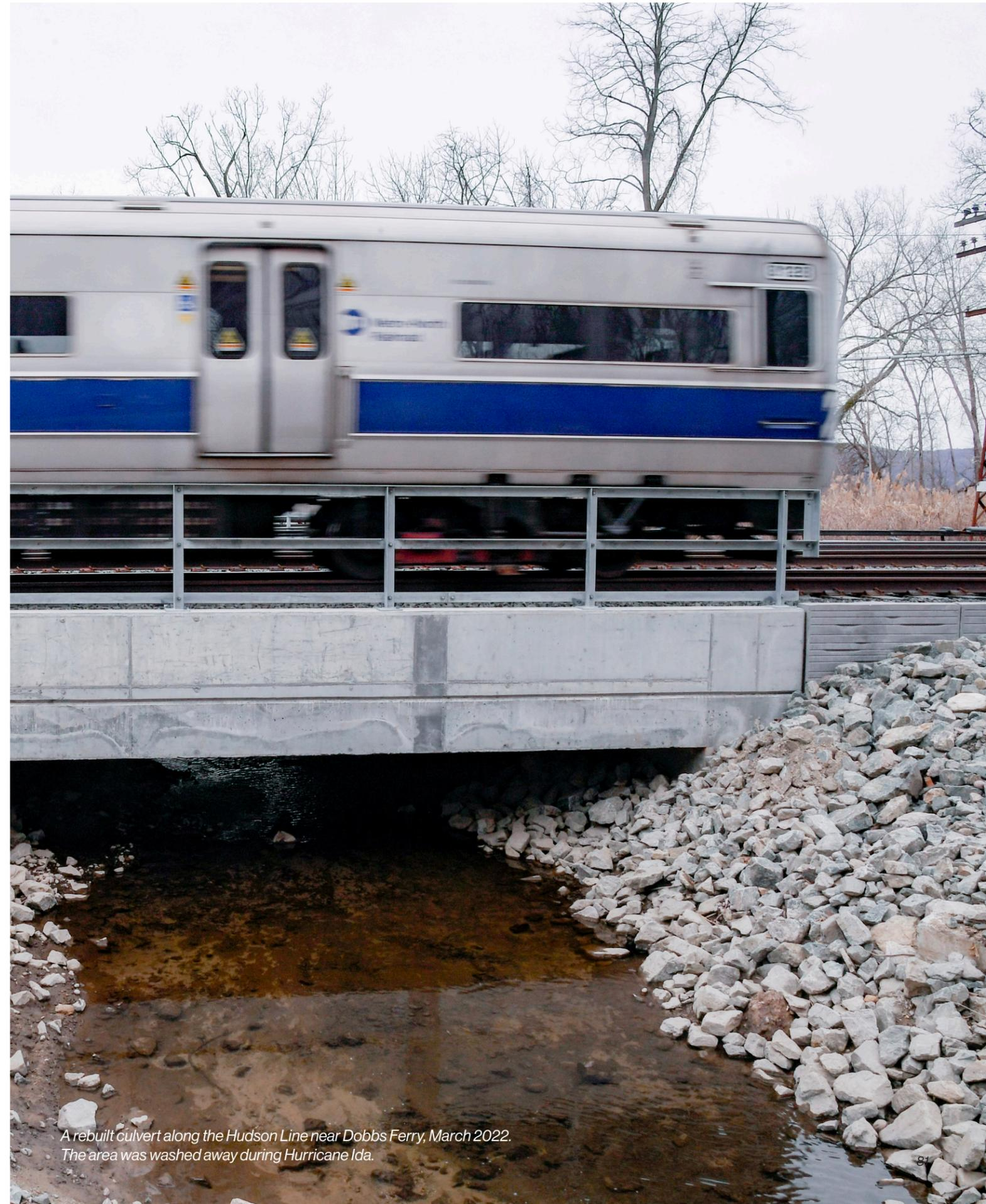
A rebuilt culvert along the Hudson Line near Dobbs Ferry, March 2022. The area was washed away during Hurricane Ida.
