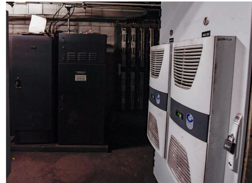
Self-cooling data cabinet in the communications room at the Wall St Station on the Lexington Avenue 4 5 Line.
