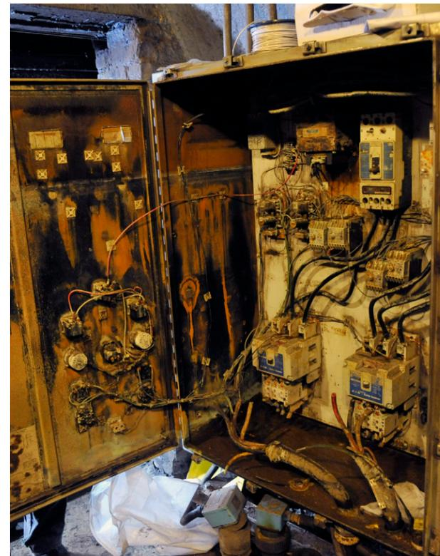
Corroded and damaged electrical circuits following Superstorm Sandy, 2012.
