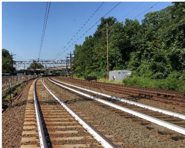
Application of heat reflective white paint along a curved section of rail near Rye on the New Haven Line.
