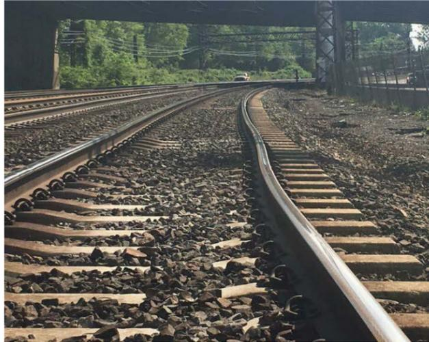
A misaligned track along the MNR New Haven Line near Rye caused by heat conditions on May 18, 2017. This progressed to a heat kink in the rail, which contributed to a derailment.
