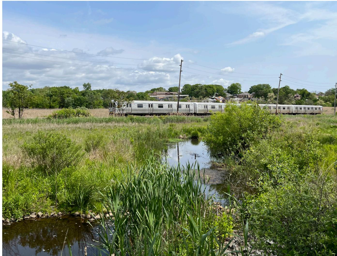
A NYCDEP Mill Creek Bluebelt retention pond south of Richmond Valley Station mitigates tidal flooding that threatens the SIR right-of-way.
