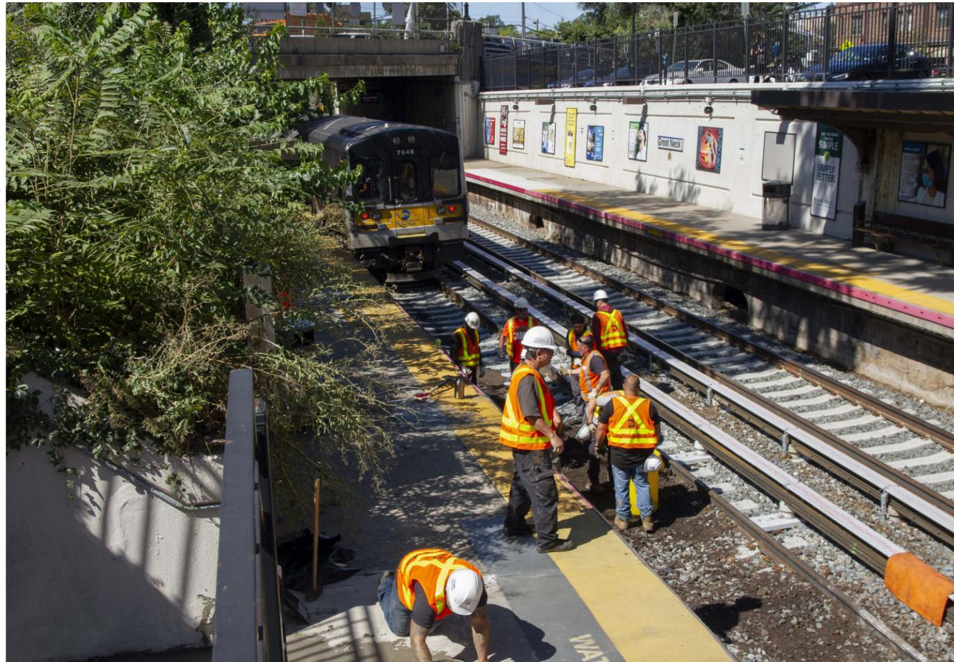
Repairs and clean-up of the Port Washington Branch Great Neck Station after Tropical Storm Ida, when torrential rainfall led floodwater and debris to cascade into the open cut right-of-way and station, impacting tracks and service.
