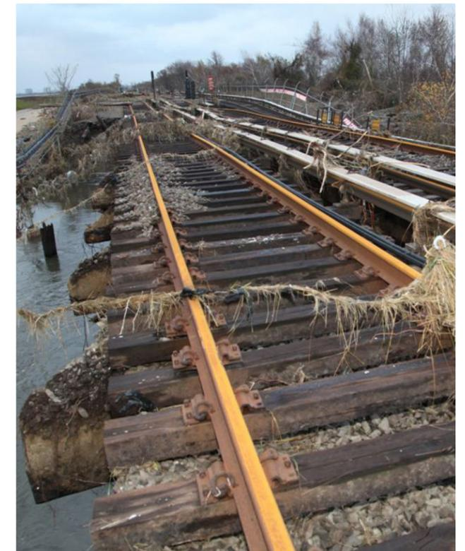
Washout, corrosion, and damage on the Rockaway Line [A](#) [S](#), following Superstorm Sandy, 2012.
