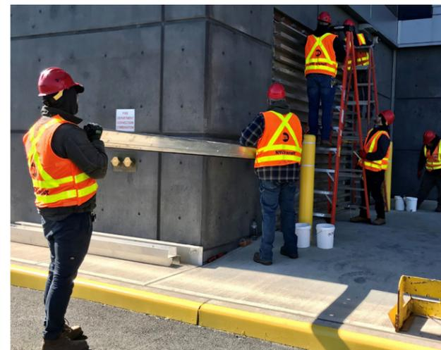
Deployment testing of flood logs at Clifton Shop, March 2023.
