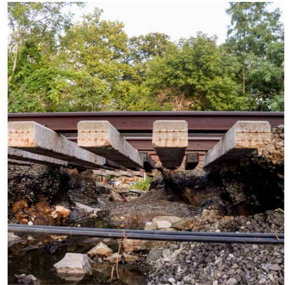
Flooding from Tropical Storm Ida washed out a culvert and the ballast supporting tracks at Dobbs Ferry, September 2021.
