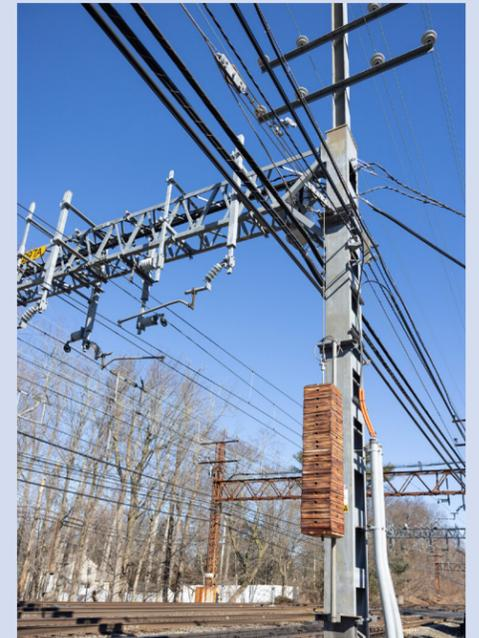
Catenary system counterweights help the system adjust to temperature fluctuations.
