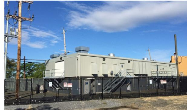
Post-Sandy, the MTA reconstructed and raised substations along the Long Beach Branch.
