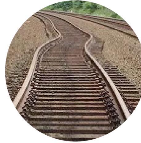
**Tracks expand**, causing buckling and misalignment. These conditions can cause service delays and speed restrictions due to safety concerns for customers and workers on trains running over compromised tracks.
