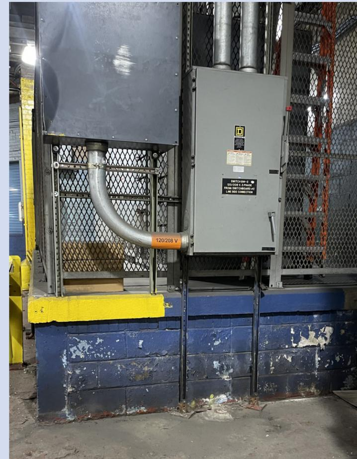
Elevated electrical equipment inside Castleton Depot. Electrical equipment in Castleton Depot is elevated above flood depth to reduce the likelihood of major damage in the event of future floods.
