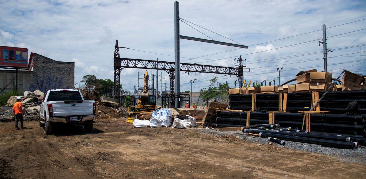
New catenary structures at Parkchester / Van Nest Station, July 2024
