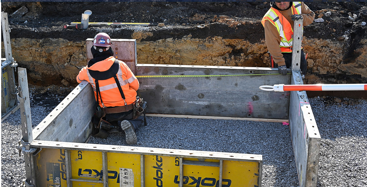
Formwork installation at Parkchester / Van Nest Substation, January 2025
