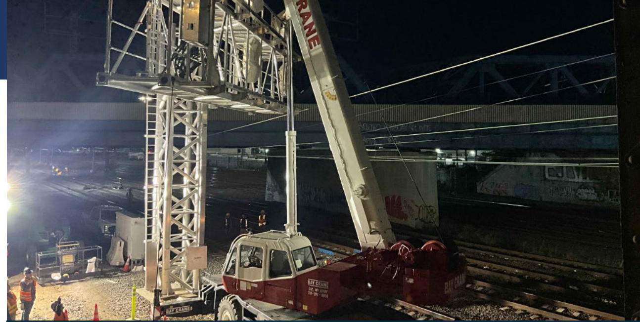
Leggett signal bridge installation, January 2025
