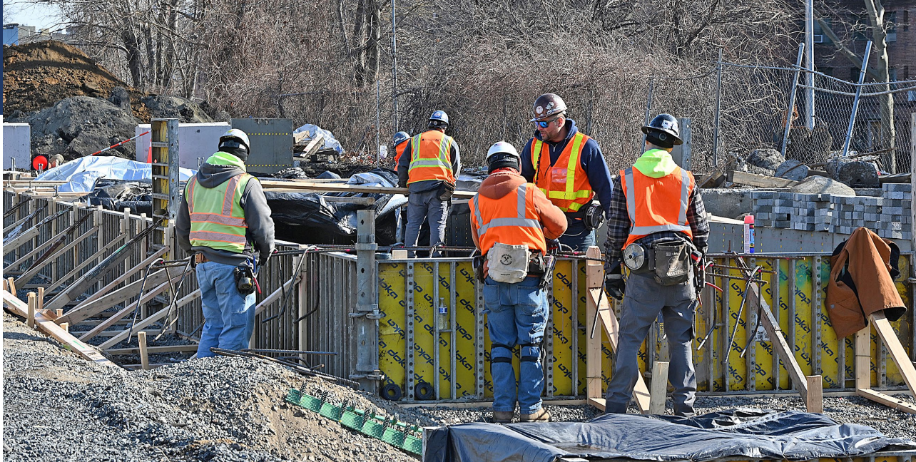
Formwork installation at Parkchester / Van Nest Substation, January 2025
