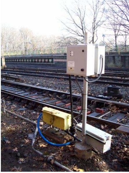
**Figure 17: New wireless controllers for Subway third rail heaters reduce costs while improving reliability**
