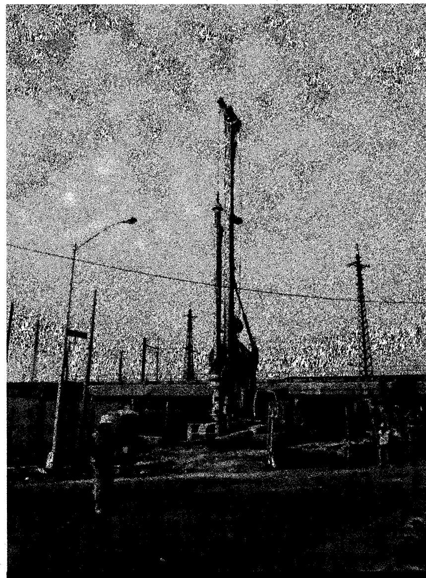
43rd Street ML4 Bridge Pier Foundation Piles (01-05-2012)
