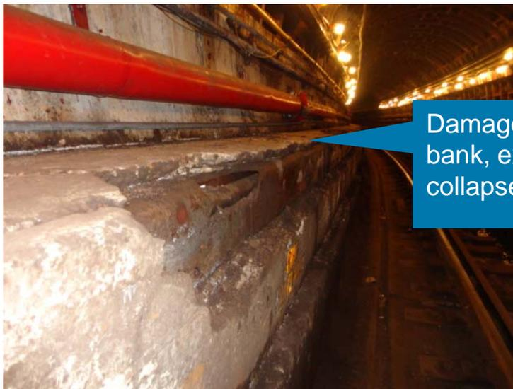
Damaged concrete bank, exposed and collapsed ducts
