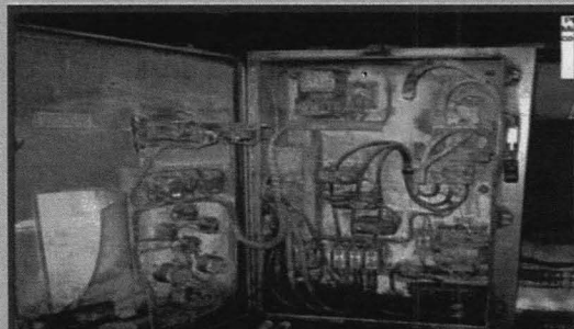
Destroyed pump control
