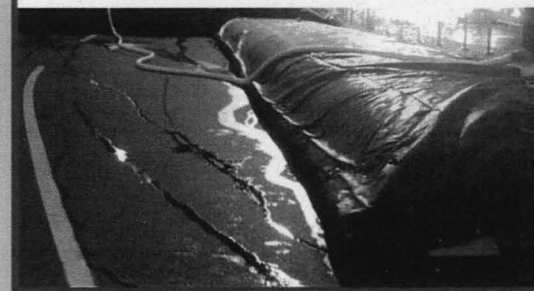
Water-filled Cofferdam
