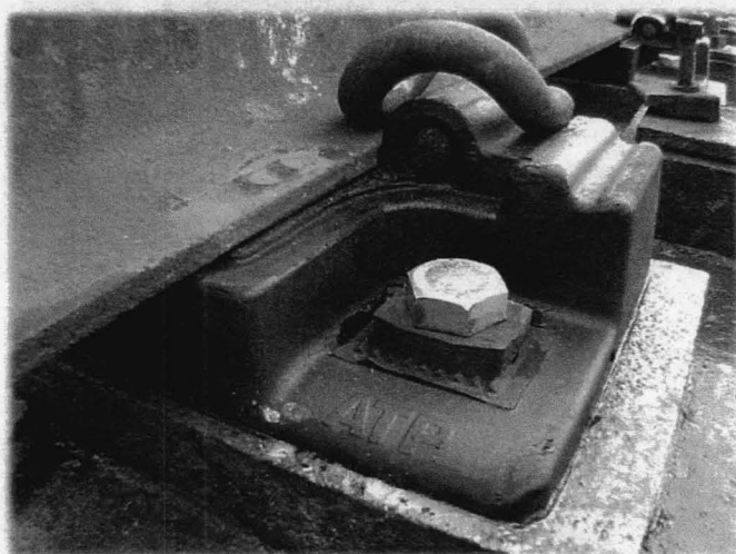
Direct Fixation Rail Fastener
