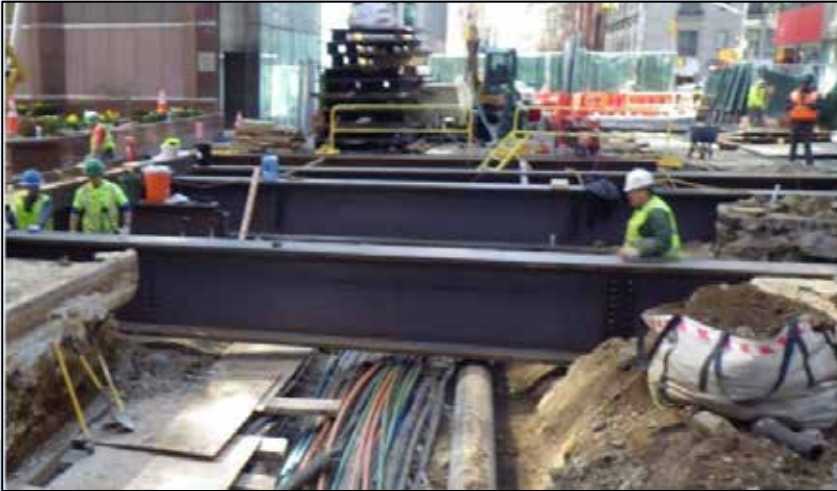
Street decking installation
