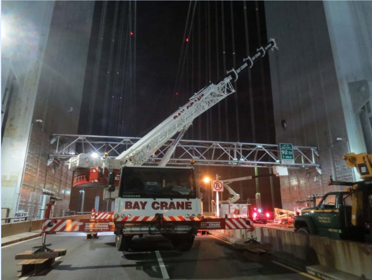
Erection of Overhead Sign Gantries at Tower Locations.
