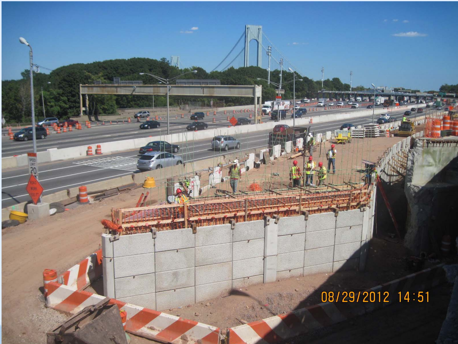
Filled structure for NRS ramp
