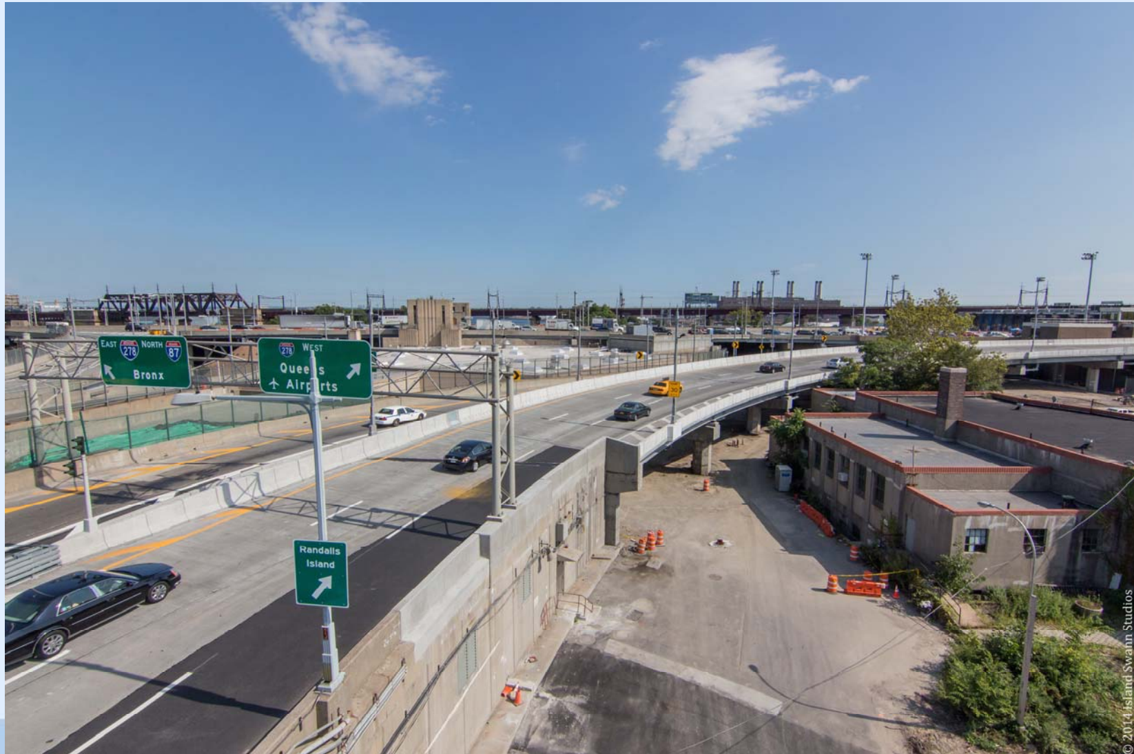
New MQ ramp deck with LED lighting
