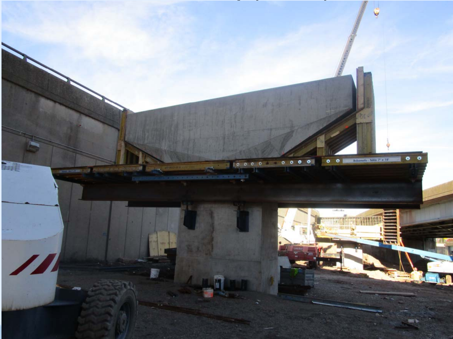
Construction of new piers for Bus/HOV Ramp
