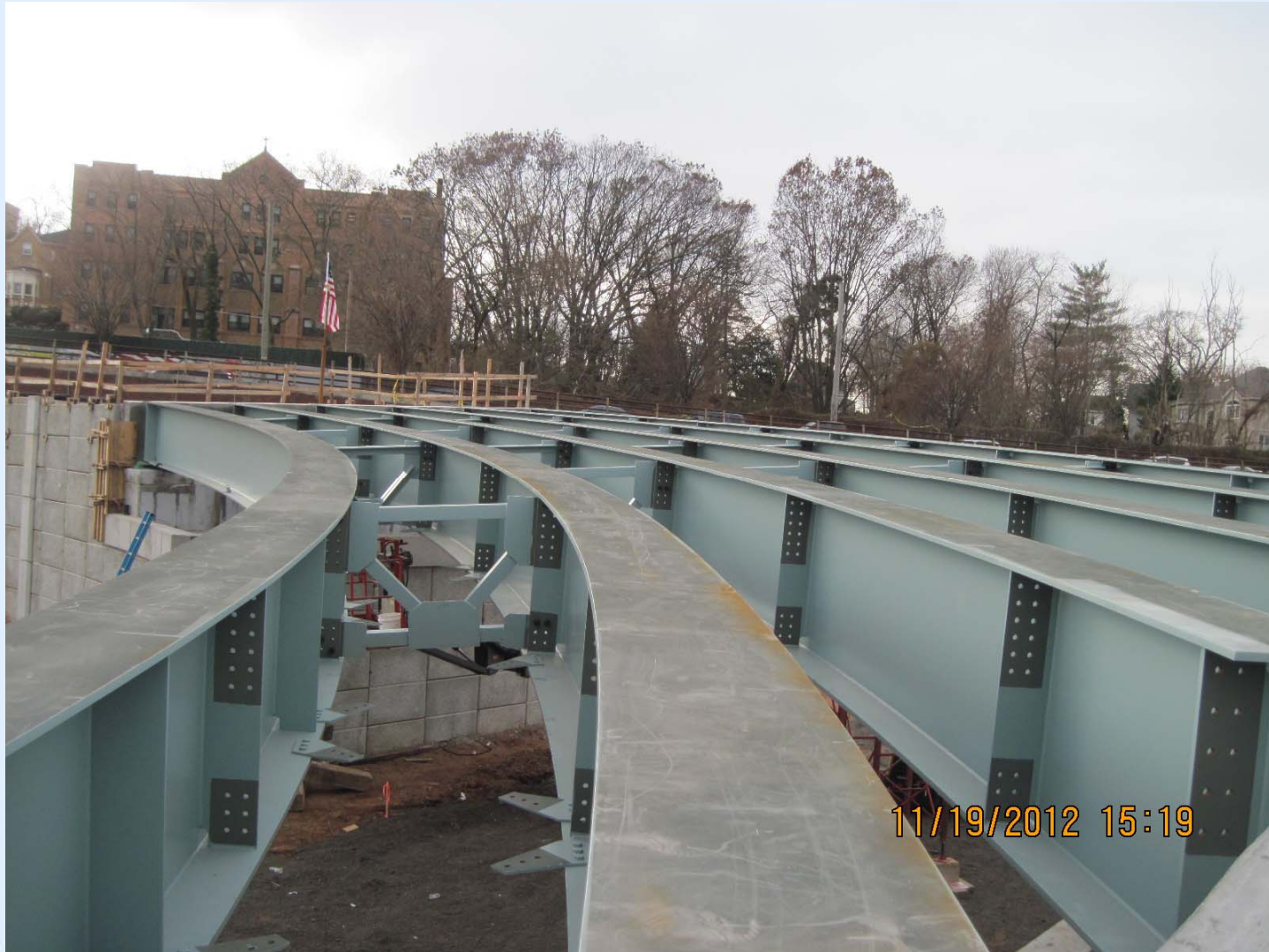
New curved steel girders for Lilly Pond Flyover Ramp
