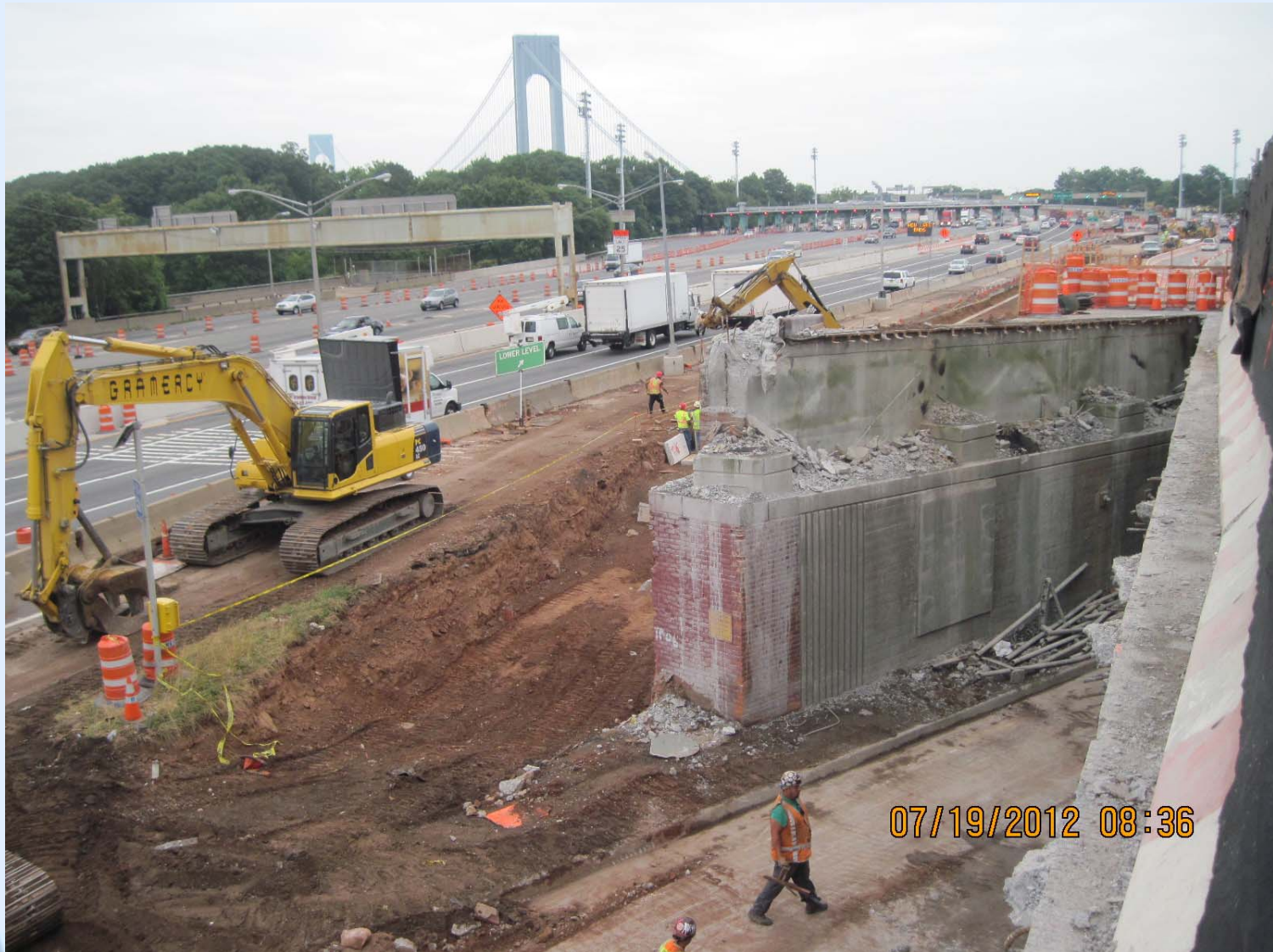
Demolition of NRS ramp
