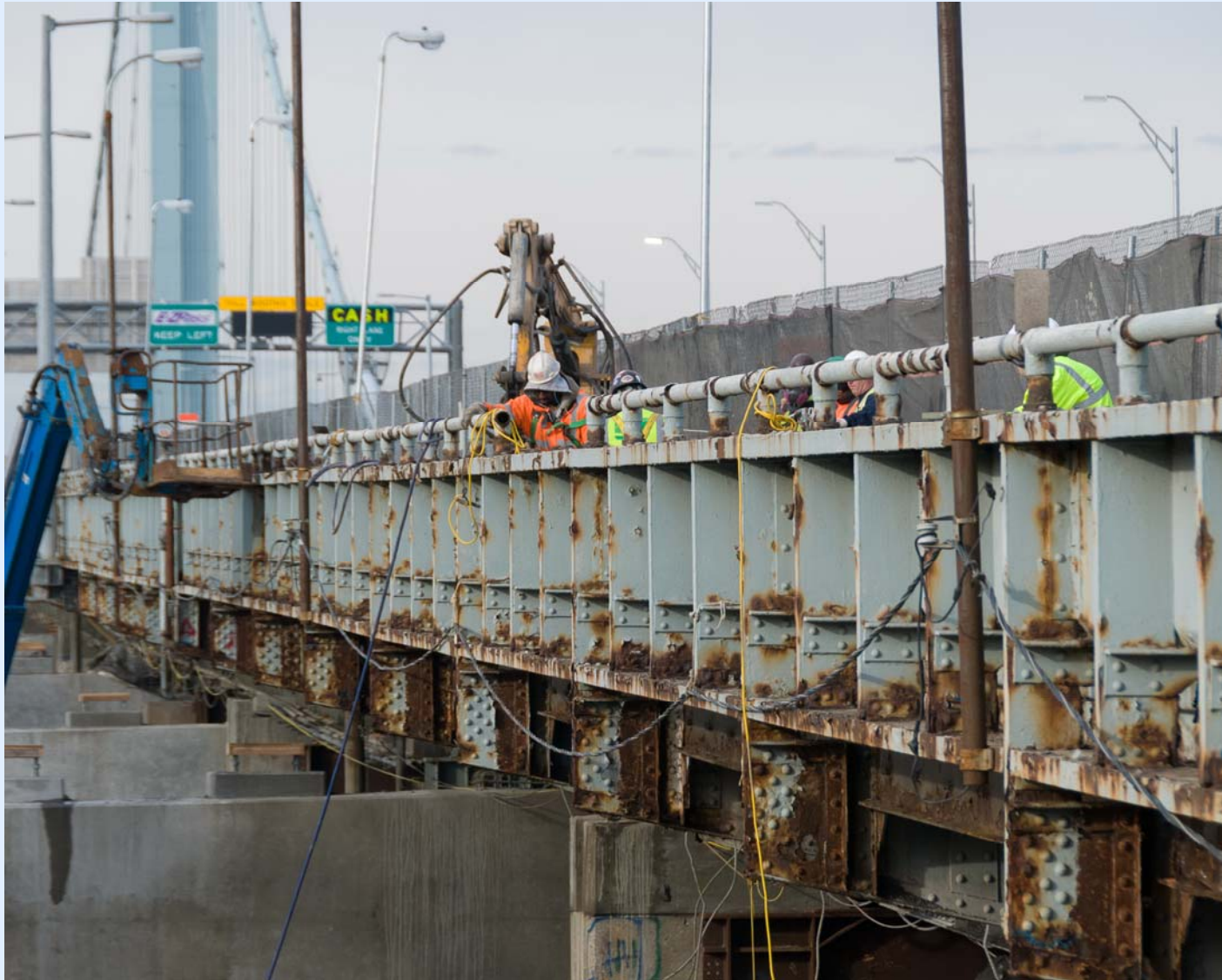
View of the Deteriorated Bridge Steel Bridges and Tunnels
