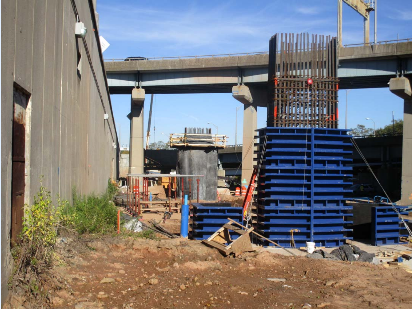
Construction of new piers for Bus/HOV Ramp
