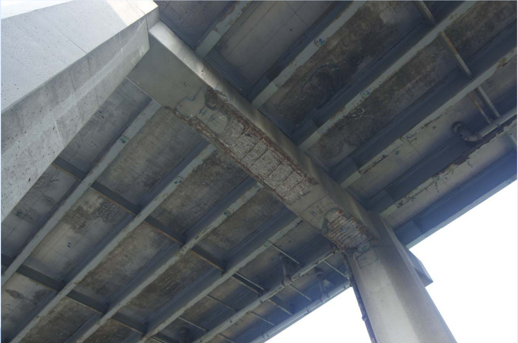
View of the deteriorated deck and pier caps
