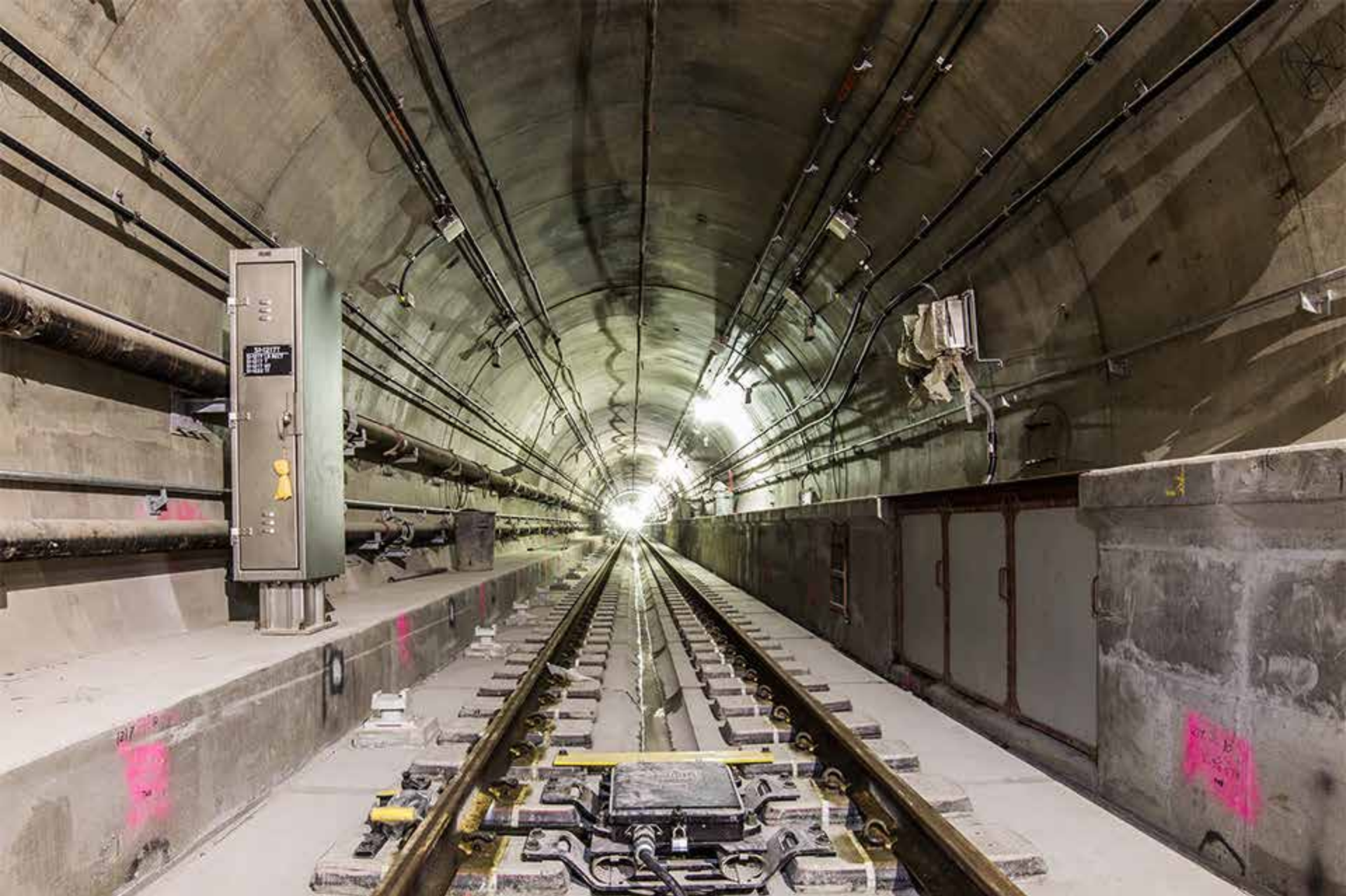
Low Vibration Track and Signal Equipment Installation – December 2014 Southbound Tunnel 86 th – 96 th Streets Looking North
