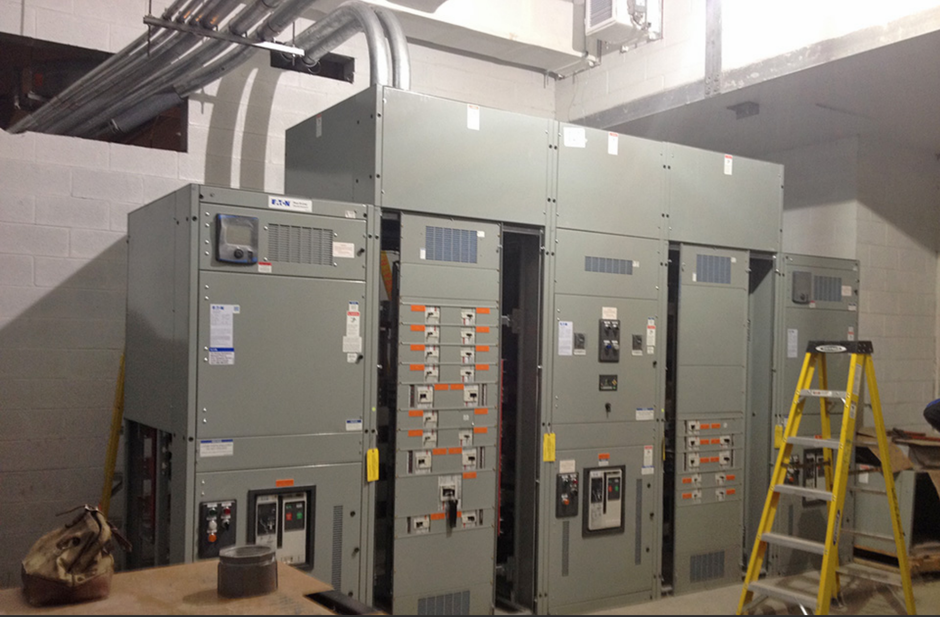
72 nd Street Station – Low Voltage Switchboard Equipment North mezzanine area
