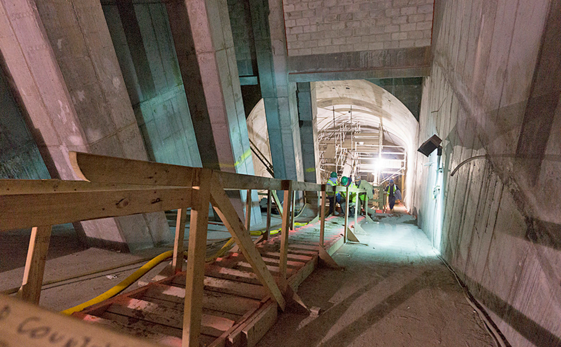
Escalator shaft through Archstone Building – January 2015
