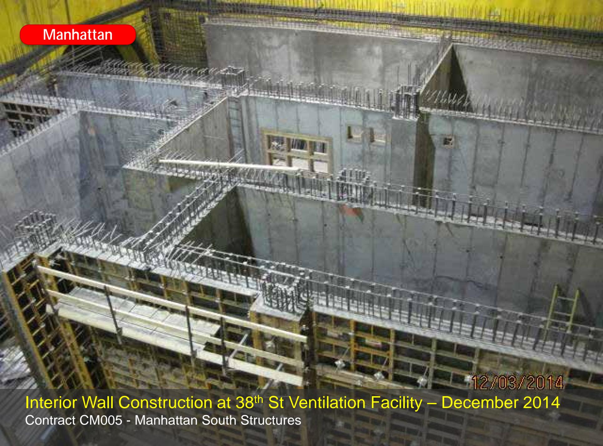
An aerial photograph showing the interior wall construction of a large facility. The walls are made of grey concrete and are surrounded by a complex network of rebar. A wooden formwork structure is visible in the foreground, and a window is visible on one of the walls. The date '12/03/2014' is printed in the bottom right corner.
