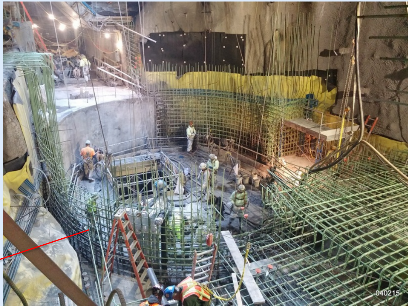
Pneumatically applied concrete for shaft final lining April 2015
