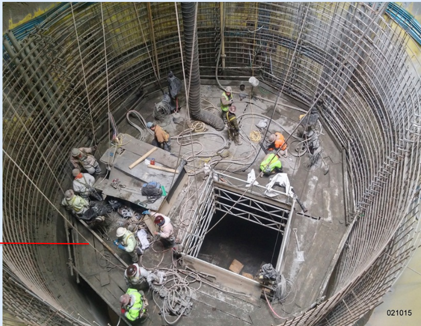
Pneumatically applied concrete for shaft final lining February 2015
