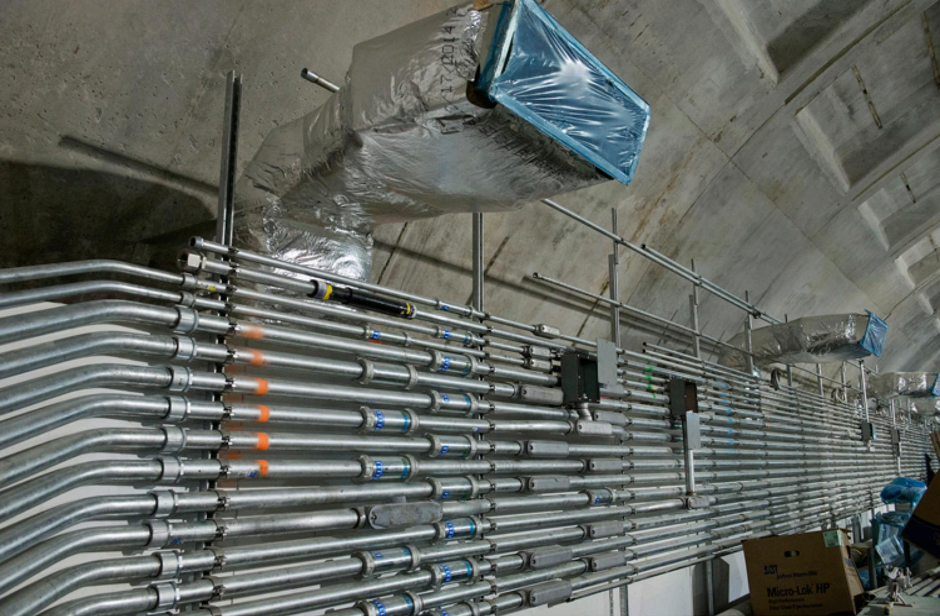
**86<sup>th</sup> Street Station** – HVAC duct work and conduit installation
