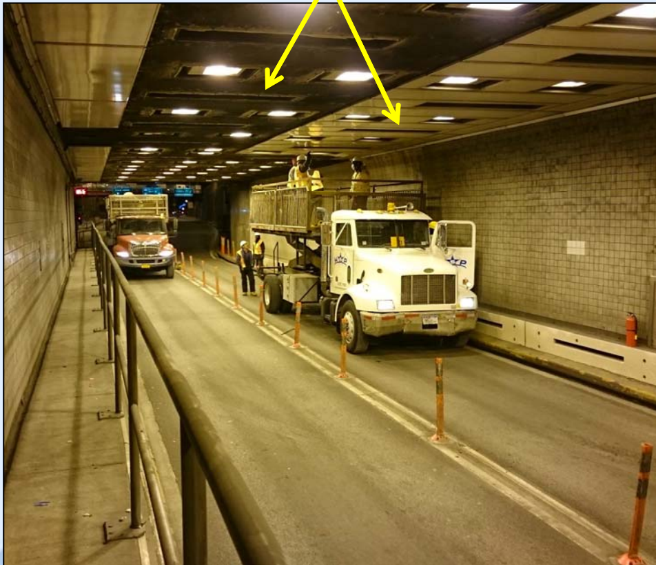
Ceiling Panel Removal at the HLCT
