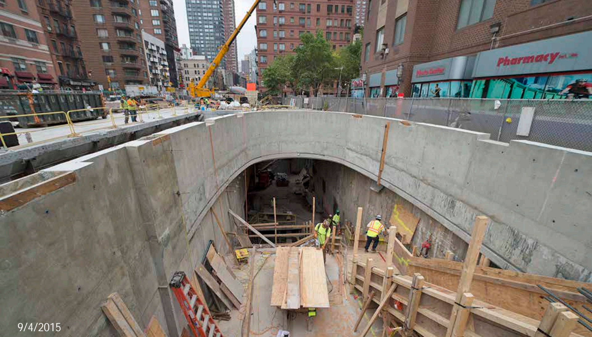
Completed Structural Shell at Entrance 3 - SW corner of 96 th Street and Second Avenue
