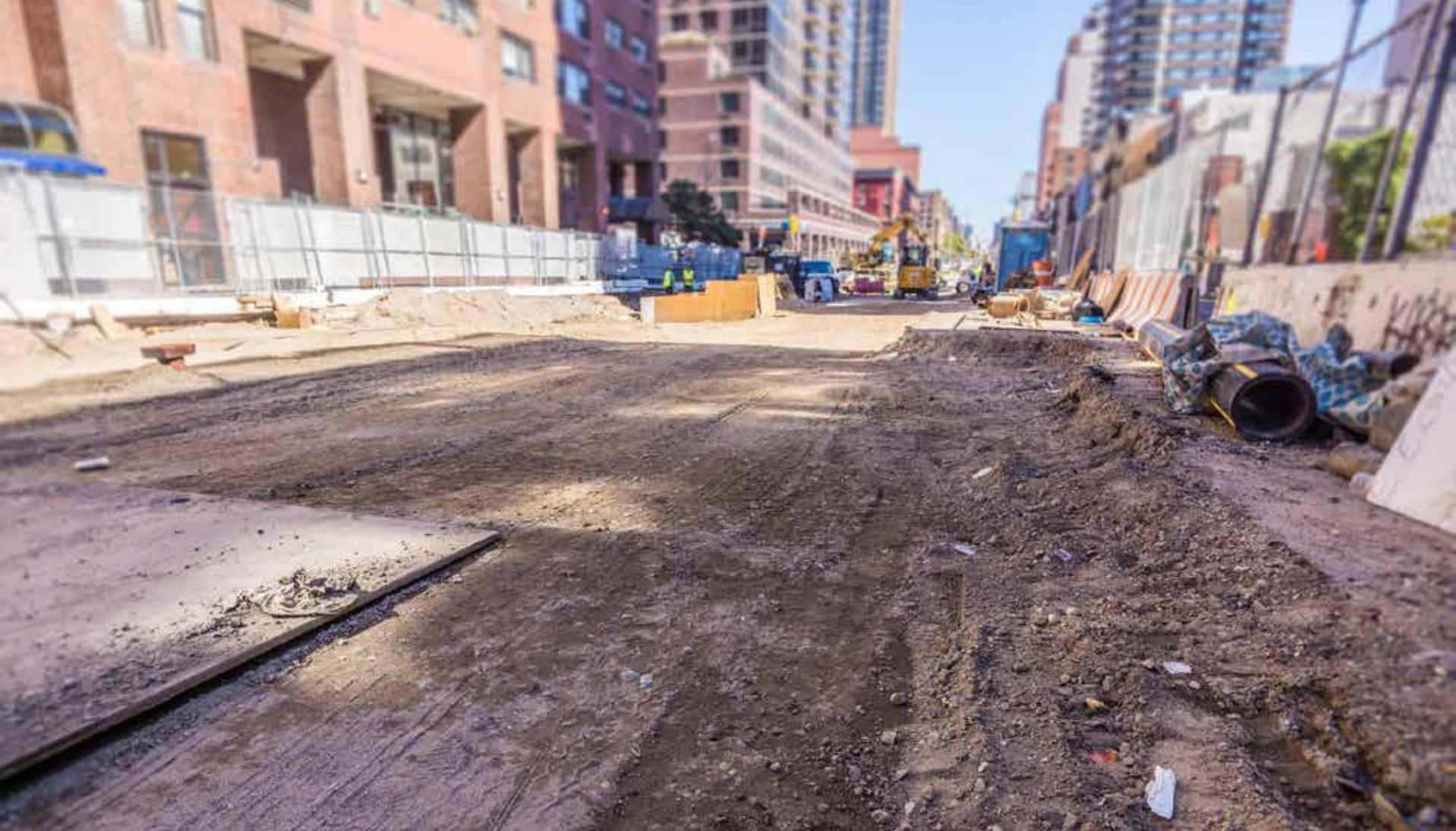
Backfill operations west side of Second Avenue, 92 nd Street looking north.
