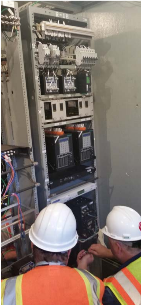
Wayside Interface Unit (WIU) Installation at CP271
