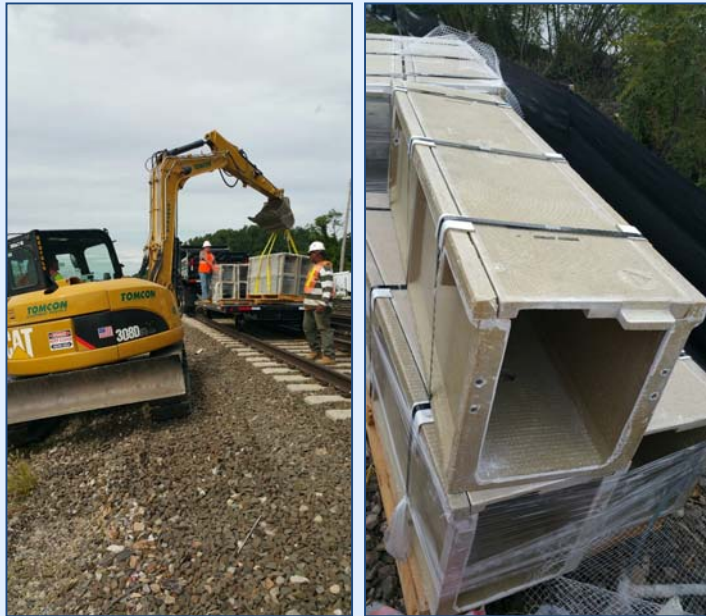
Work in progress – Installation of Cable Trough
