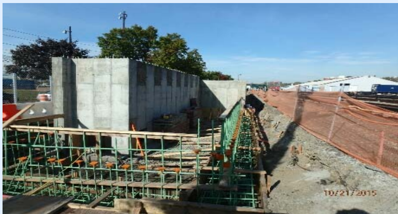
Work in progress – Substation foundation
