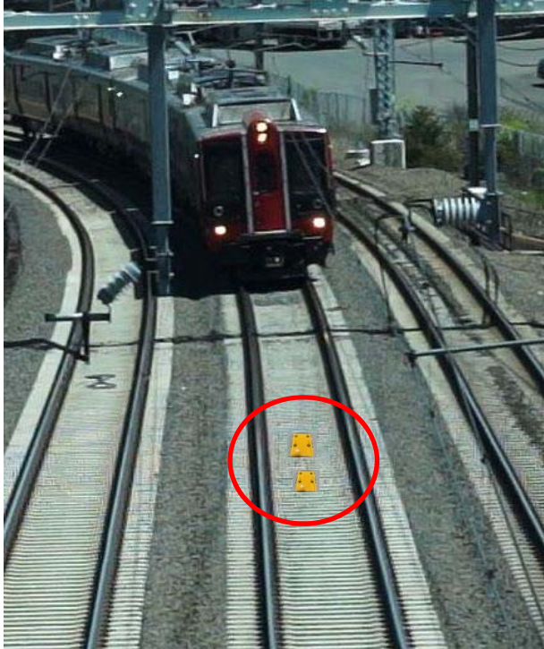
Transponders installed between the rails on the New Haven Line
