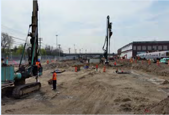
Consist Shop facility concrete floor slabs, excavations and installation of electrical duct banks, water and storm drains utilities.
