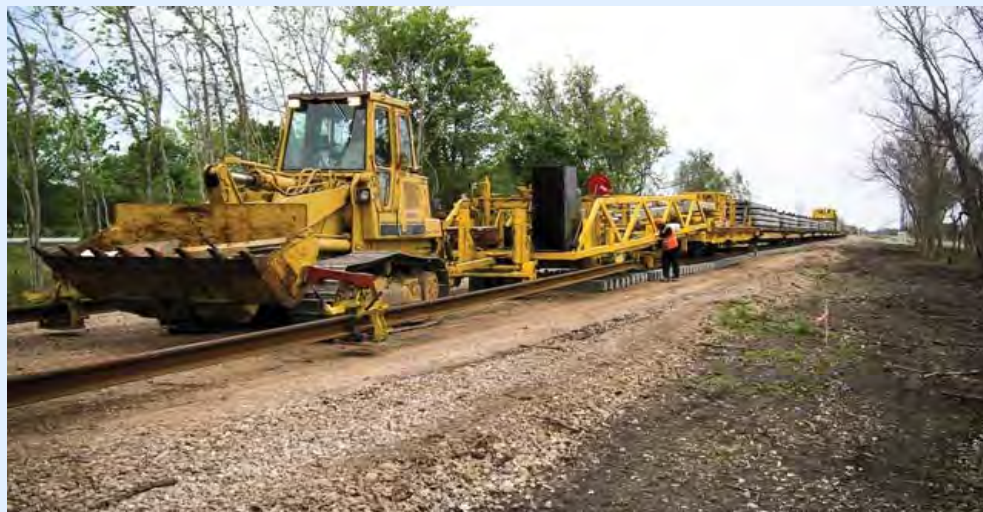
New Mechanized Track Installation
