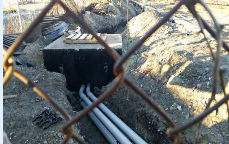
Signal Power Conduit / Manhole installed
