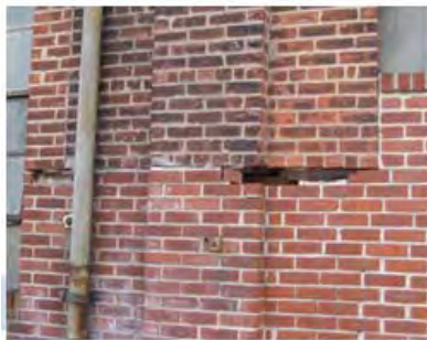
Cracks and Voids
