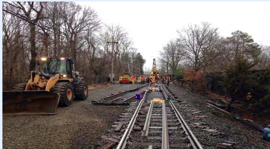
New Switch Installations
