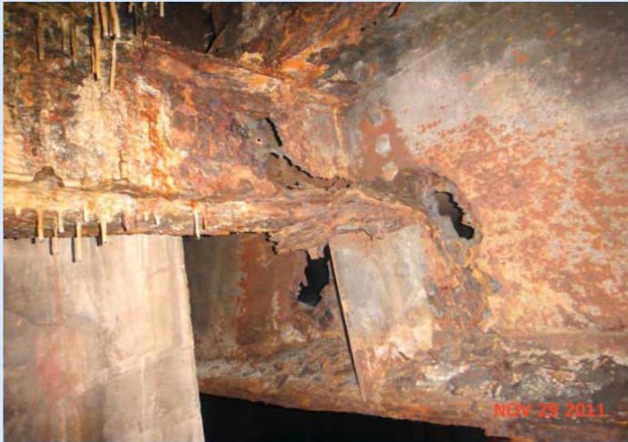
Prior condition of a structural steel member as a result of water seepage
