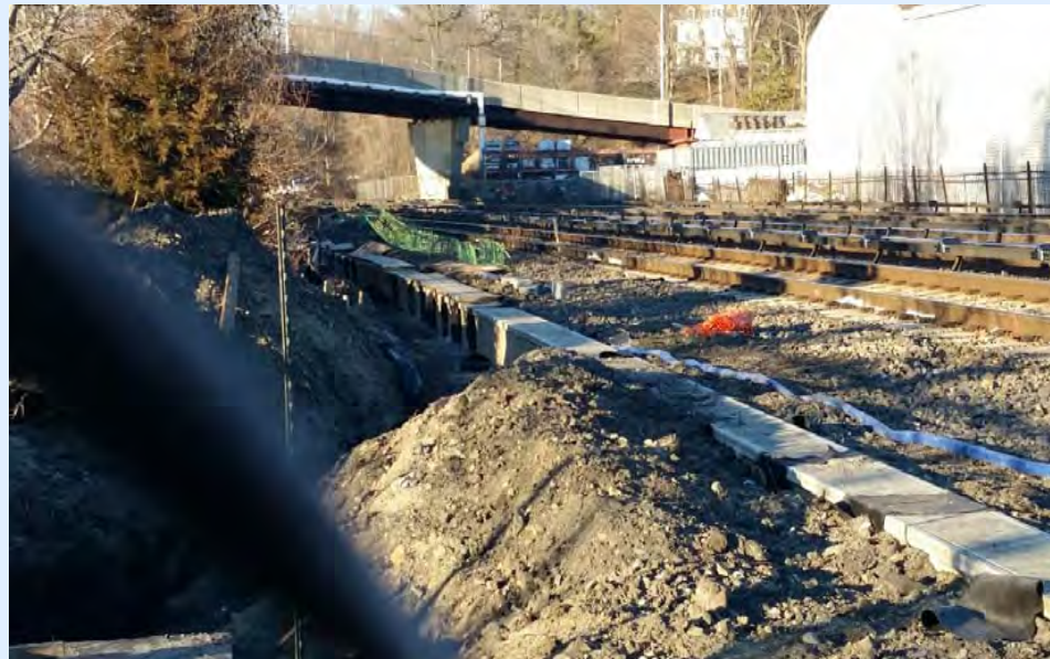
C&S Trough installation
