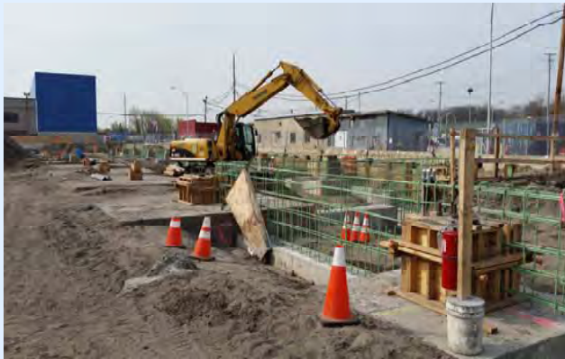
Installation of formwork, rebar and foundations at the EMU (Electric Multiple Unit) Annex.
