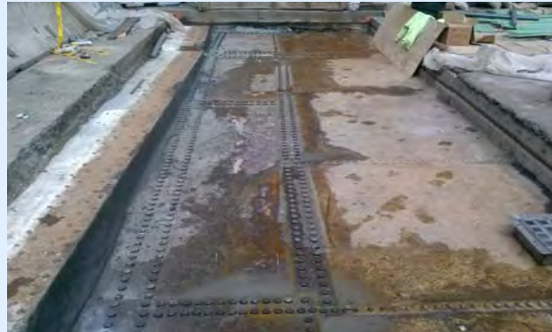
Restored structural steel at 42 nd Street and Vanderbilt Avenue
