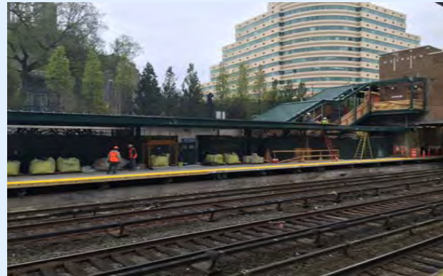
Platform Canopy installation in-progress on Outbound Platform 80% Complete
