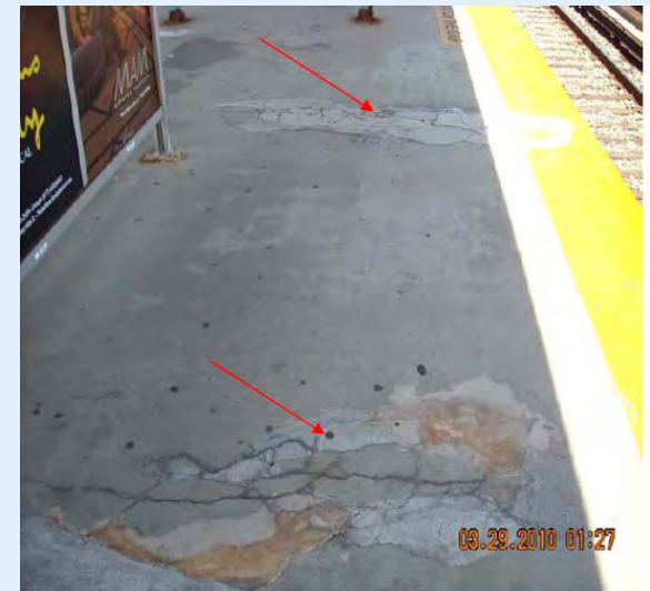
Deteriorated & Spalled Concrete Platform
