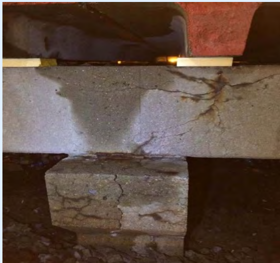
Deteriorated Platform Substructure
