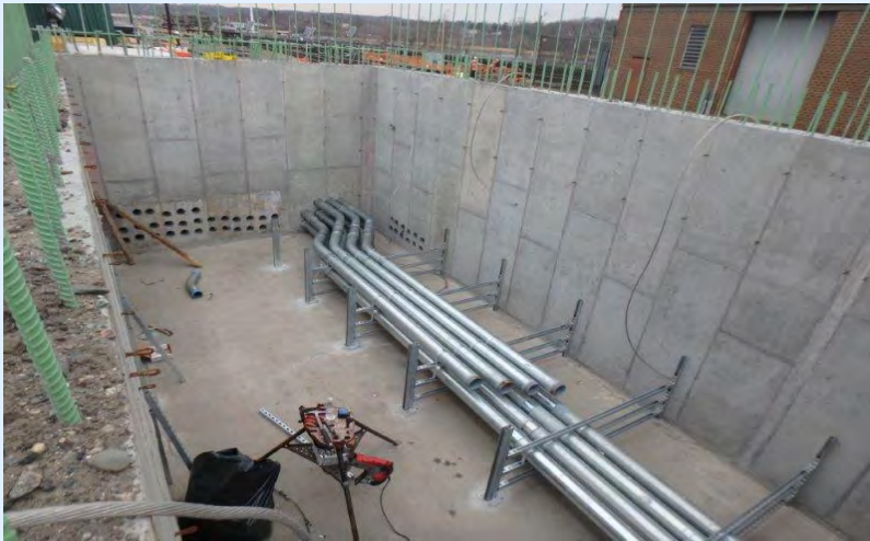
Elevated vault foundation for new A-33 Harmon Substation
