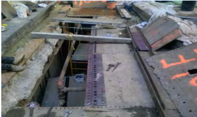
Demolition of deteriorated structural steel due to leaks at 42 nd Street and Vanderbilt Avenue
