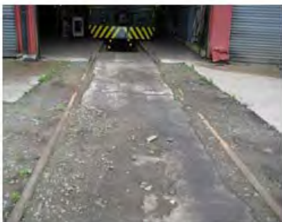
Sinking Tracks Leading Into Shop
