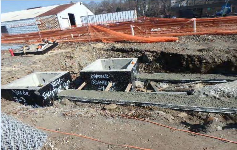
Concrete Placement for Duct Banks
