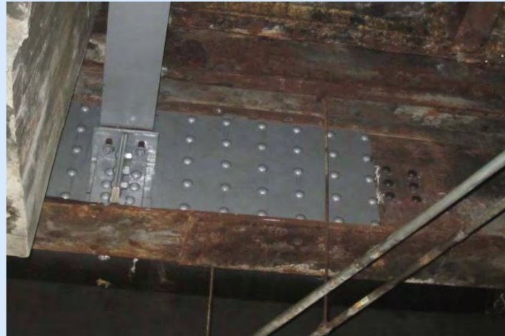
Repaired structural steel member
