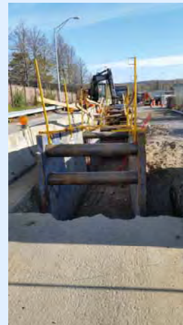
Excavation and installation of medium voltage (13.2Kv) and communication duct banks and manholes.
