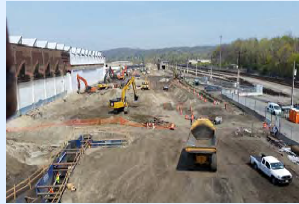
Installation of compacted aggregate piers for the Consist Shop foundations at north end.
