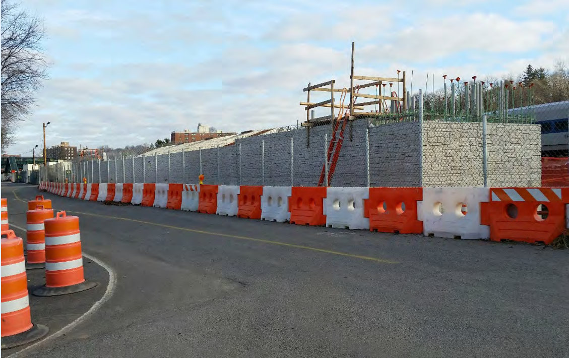
Elevated vault foundation for new A-25 Tarrytown substation
