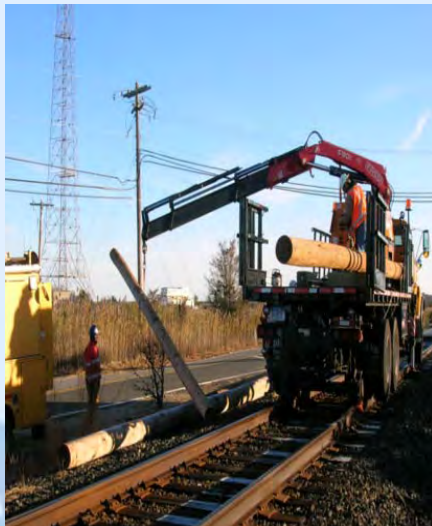
Pole Replacement Preparation
