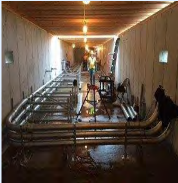
Elevated vault foundation for new A-13 Riverdale Substation
