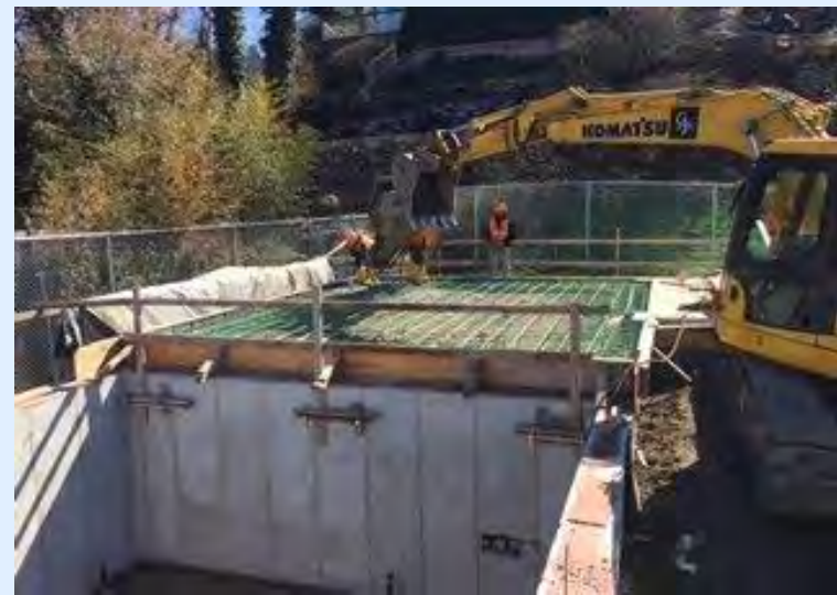
Foundation for new crew quarters adjacent to A-13 Riverdale Substation
