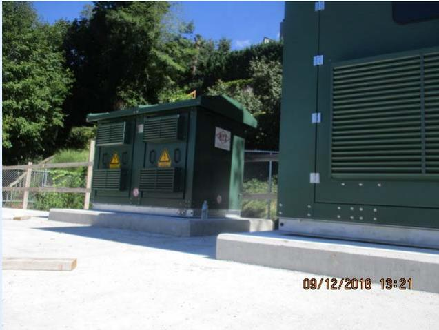
*New 2.3MVA Rectifier , and 112.5 KVA
