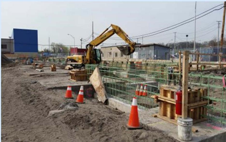
*May 2016 – Installation of formwork, rebar and foundation at the EMU (Electric Multiple Unit) Annex.*
