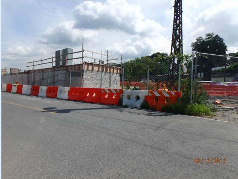
Elevated vault foundation for new A-25 Tarrytown substation
