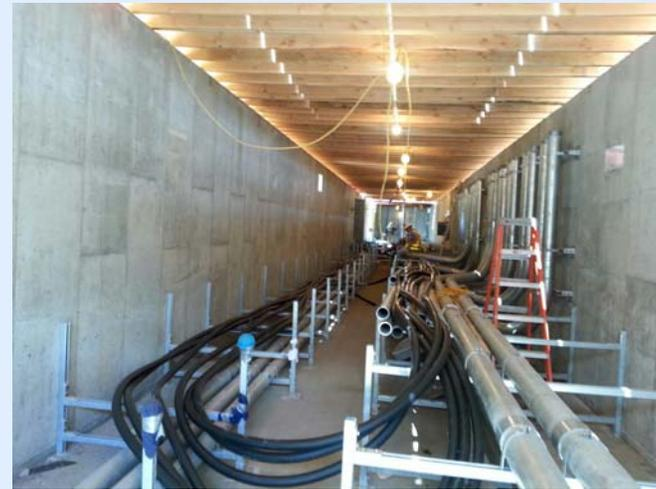
*Elevated vault foundation for new A-33 Harmon Substation*
