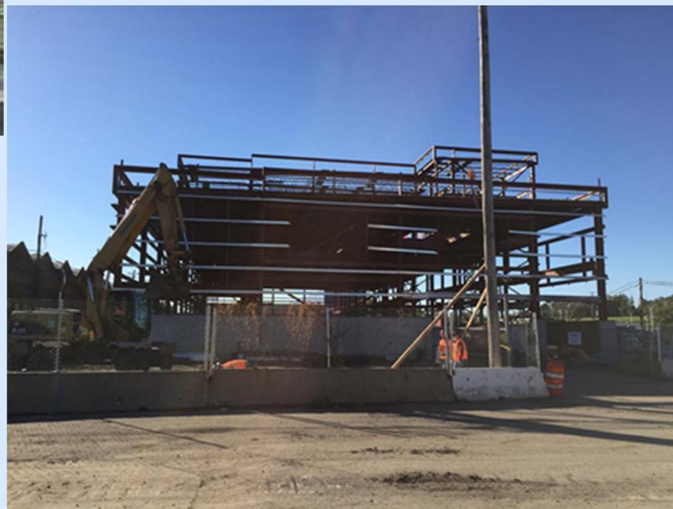
*October 2016 – Installation of Structural steel completed at the EMU Annex, in-slab utilities on 2<sup>nd</sup> floor on progress.*
