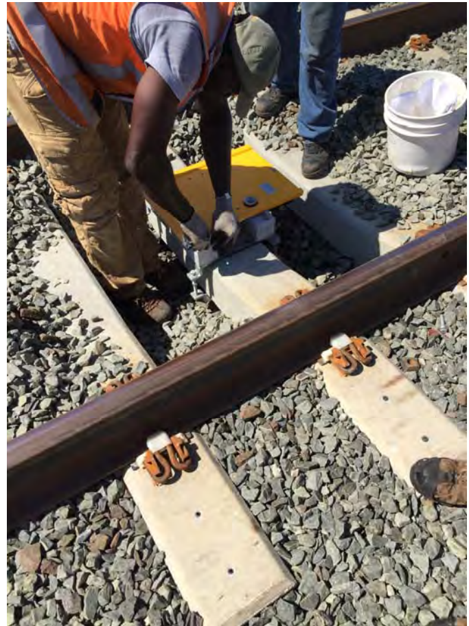
Transponders Installation on Concrete Tie
