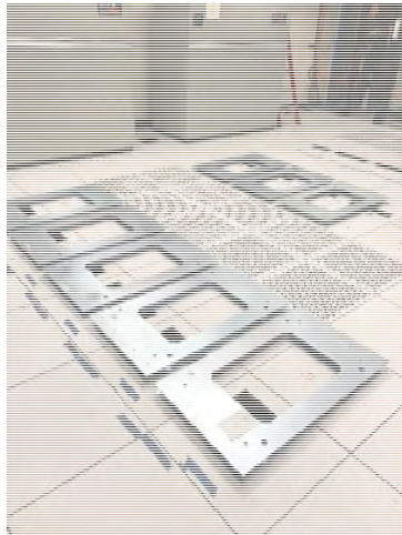
Isolator Plate Install in the Back-up Control Center (BCC)
