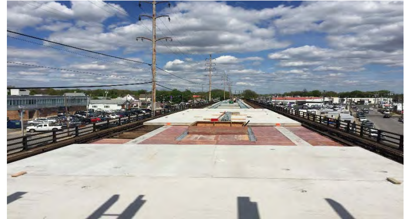
Precast Platform Slab
