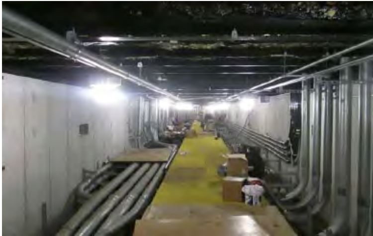
RIVERDALE: Fiberglass Raised Platform in Vault
