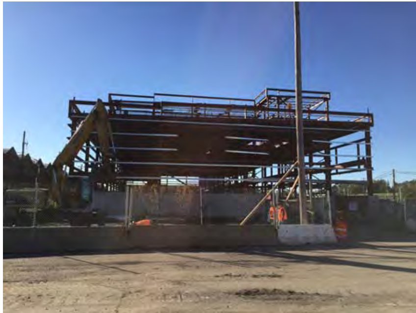
October 2016 – Installation of Structural steel completed at the EMU Annex , in-slab utilities on 2 nd floor in progress.
