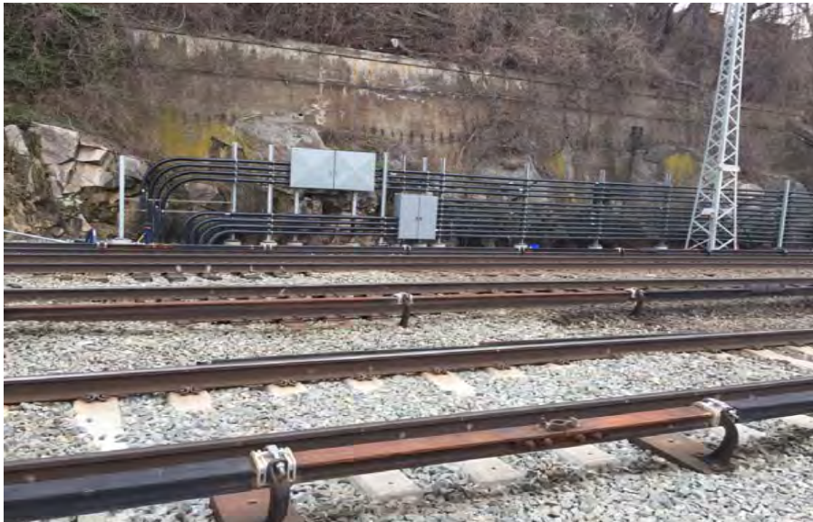
Conduit and Cable installation along East Wall at Ossining
