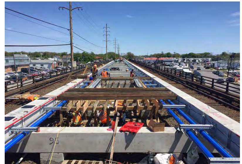
Substructure with Formwork – Track Level
