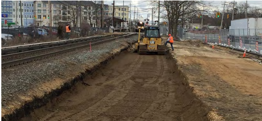
Trackbed excavation at Wyandanch
