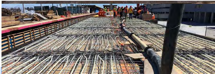
Form/Piping for New Platform
