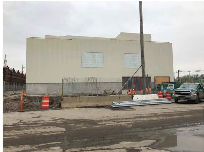
May 2017 – Installation of insulated metal wall panels and Kalwall translucent wall panels completed. Installation of roofing, MEP utilities, CMU walls, painting and stairs are ongoing. Delivery of Mechanical and Electrical equipment has commenced.
