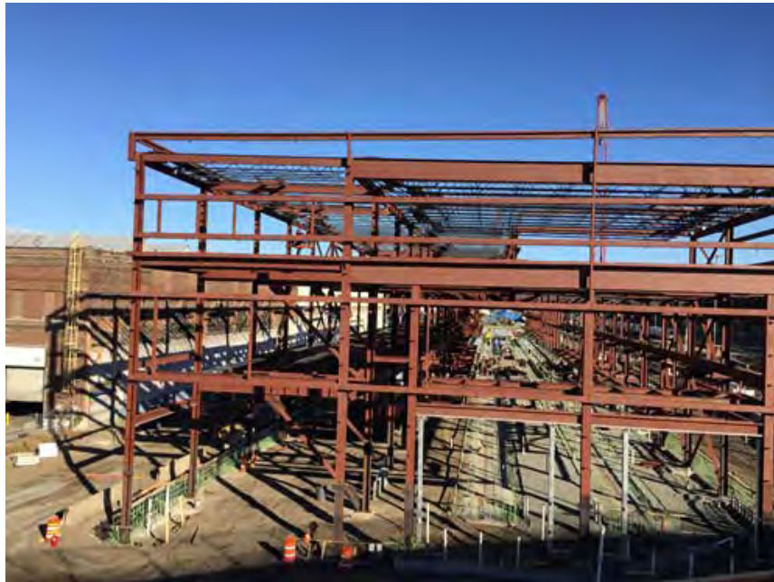
October 2016 – Installation of Consist Shop Facility structural steel, floor slabs, foundation walls, and track pits.
