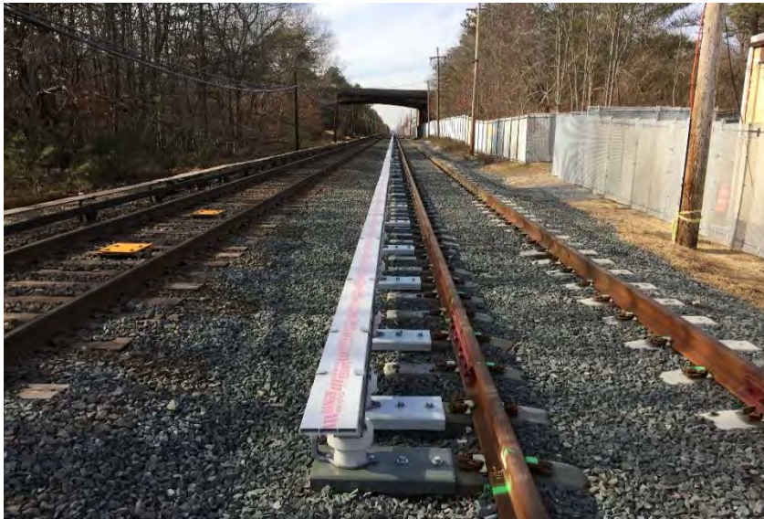
Third Rail Installation by Force Account
