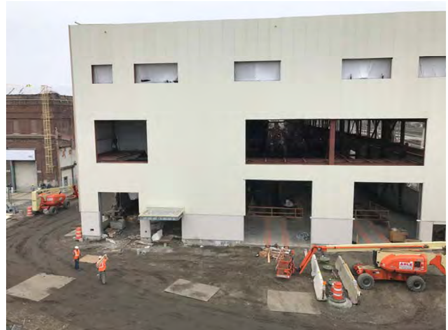
May 2017 – Consist Shop Facility – Installation of Precast perimeter walls, insulated metal wall panels complete. CMU walls, MEP utilities, roofing, painting and elevated track rail installations are ongoing.
