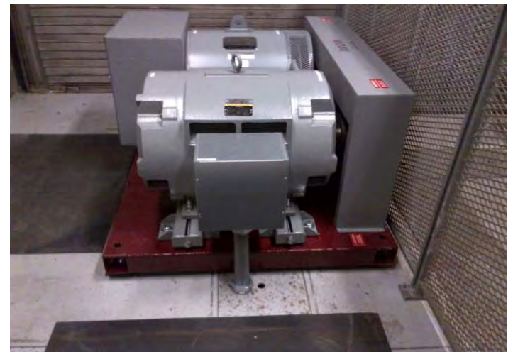
Signal Power Motor-Generator
