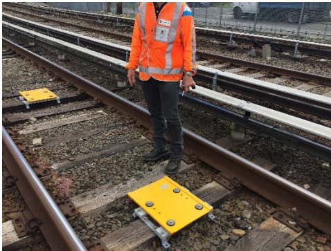
Transponders Installation on Far Rockaway Branch
