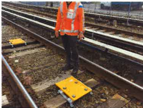
Transponders Installation on Far Rockaway Branch
