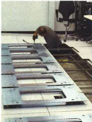
Office PCC Isolator Plate Installation
