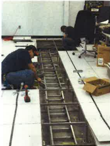
Primary Computer Center (PCC) Cable Tray Installation
