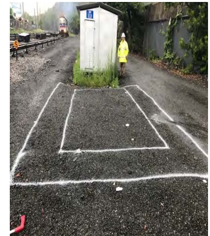
Utility locate mark out Phase II
