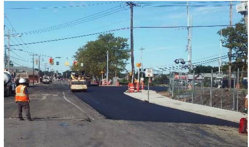
New paving at grade crossing in Wyandanch
