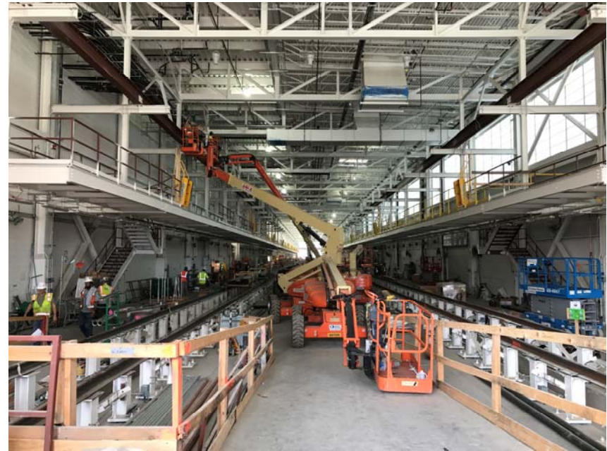
September 2017 – Building envelop is nearing completion. CMU walls are complete, Roof level platforms and track rail installations are complete. MEP utilities, painting, and HVAC ongoing.
