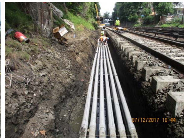
4" PVC conduits installation at North of Philipse Manor
