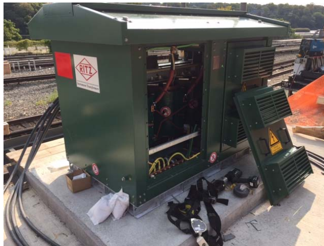
CROTON-HARMON: Termination of Cables at Transformer
