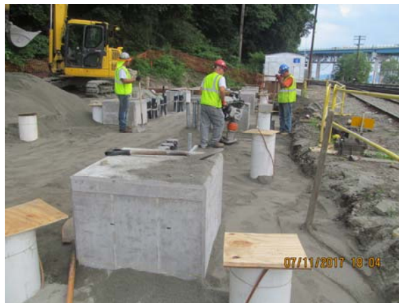
Backfill with Sand - Platform foundations at Tarrytown
