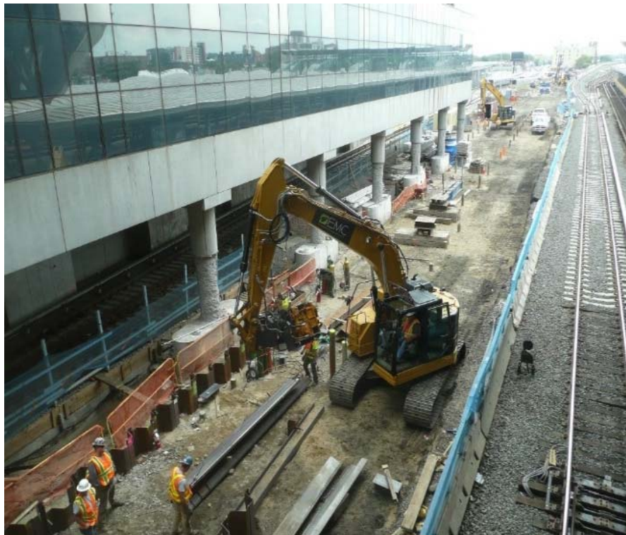
Support of Excavation – Future Platform F Stairway
