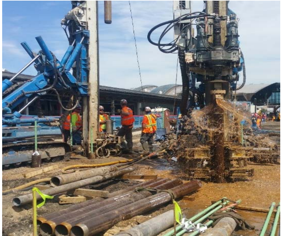
Pile Drilling - Future Platform F
