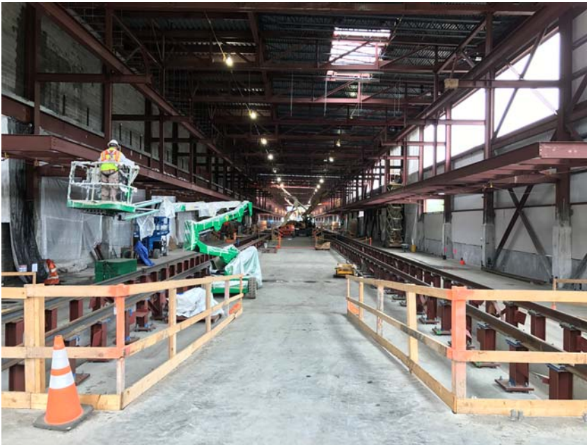
May 2017 – Consist Shop Facility : Installation of car roof level platform railings and stairs, and preparation for translucent wall panels, roof skylights and interior painting.
