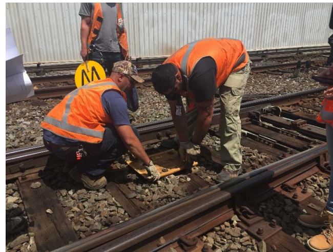
Pilot Line 1 Transponder Installation
