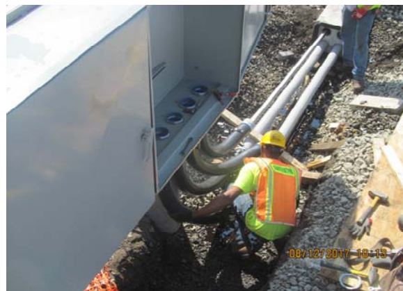
Signal pull box south of Croton Platform between Track 1 & 2
