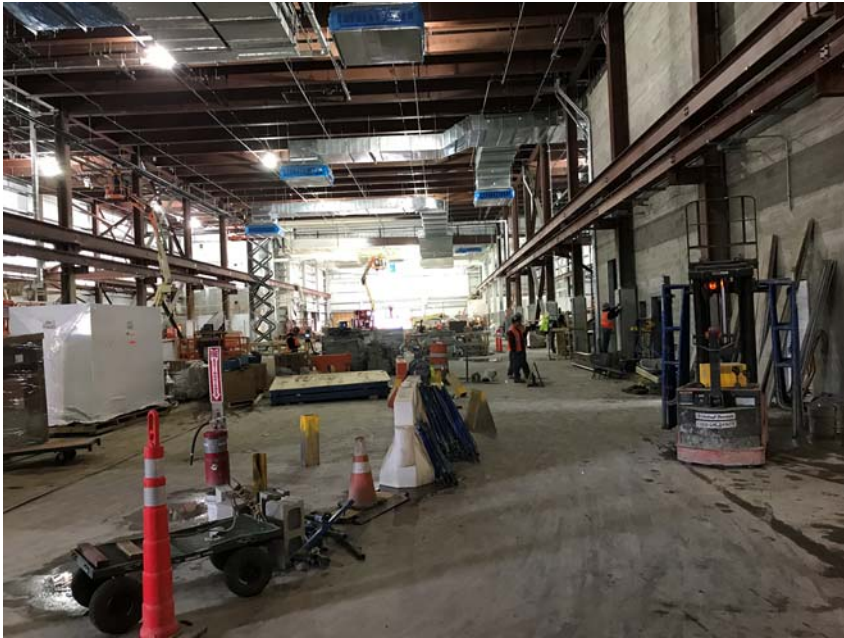
May 2017 – EMU Annex : Installation of MEP utilities underway, delivery of mechanical, electrical and elevator equipment and preparation for interior painting.
