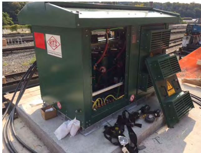
CROTON-HARMON: Termination of Cables at Transformer
