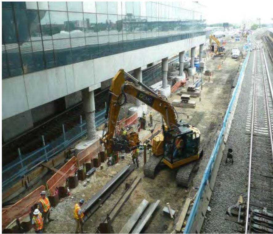
Support of Excavation – Future Platform F Stairway
