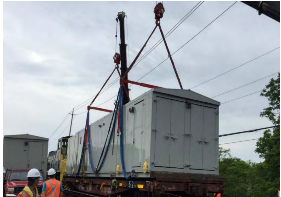
Phase 1: Setting of CI (Central Islip) Interlocking Hut
