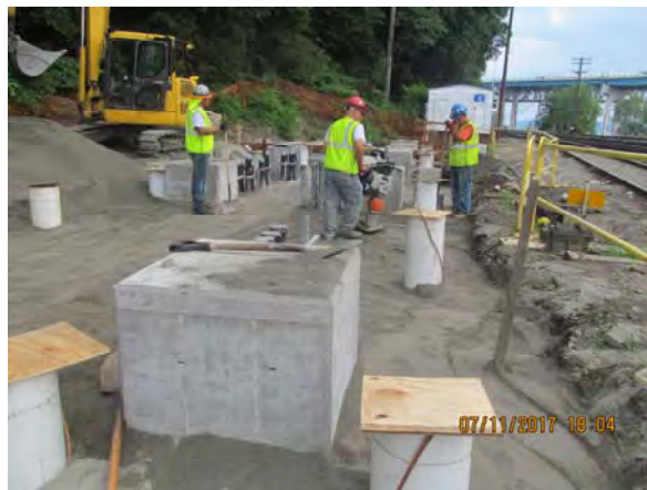
Backfill with Sand - Platform foundations at Tarrytown
