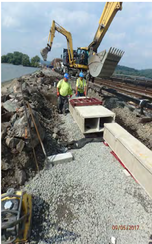
Installation of Double trough at Croton River Causeway
