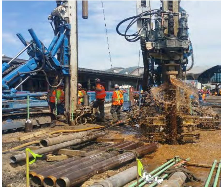
Pile Drilling - Future Platform F
