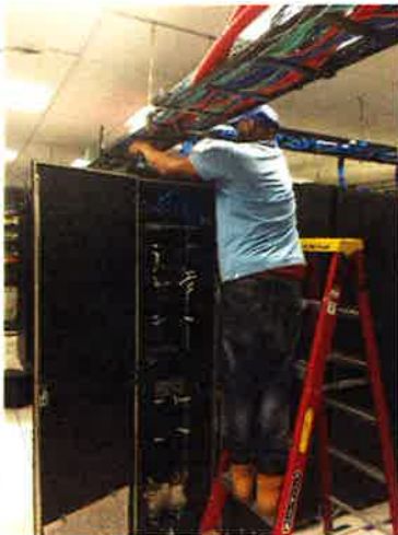
BCC Office Patch Cable Installation
