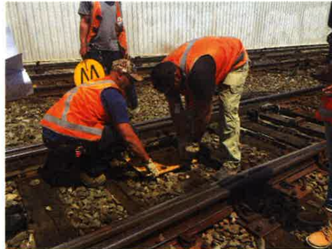
Pilot Line 1 Transponder Installation
