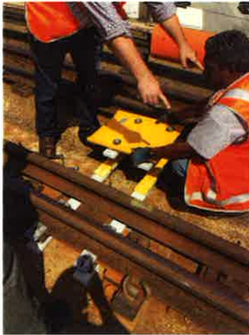
Vortok Bracket Trial Installation
