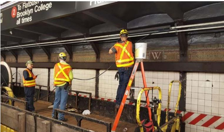
Fiber Optic Cable Installation
