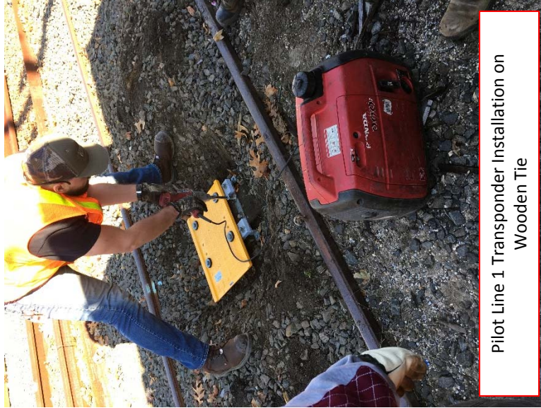
Measurement of Transponder Install Location on Pilot Line 1
