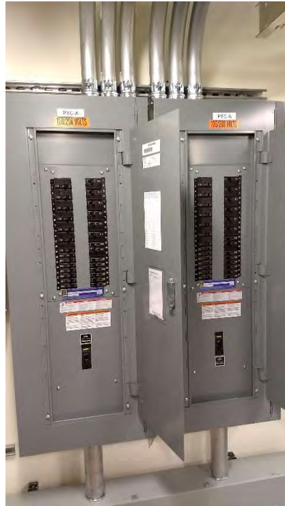
Conduit/Electrical service/Office Equipment installed at the Emergency Control Center (ECC)
