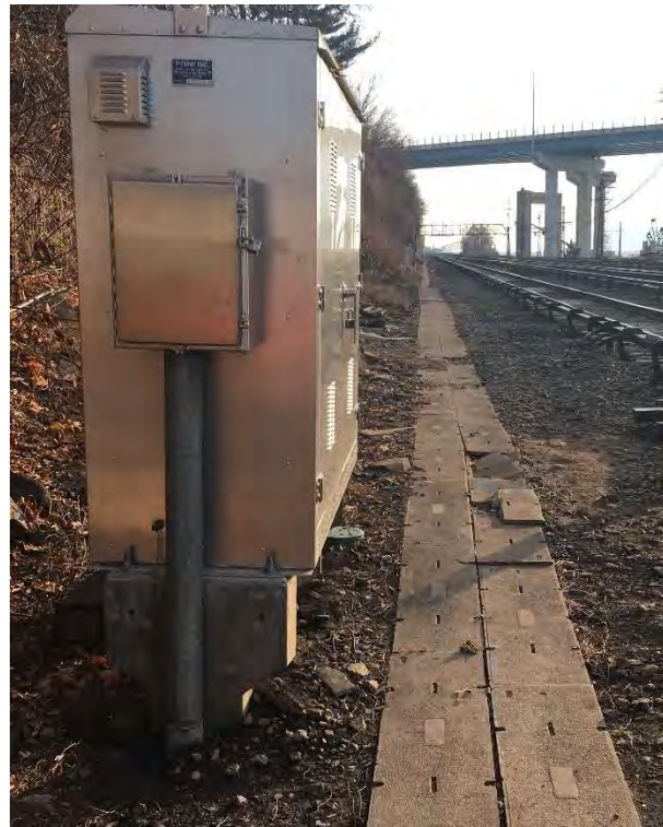
Antenna Pole/Radio Case/Communication Interface Case Installed at Tarrytown CP25
