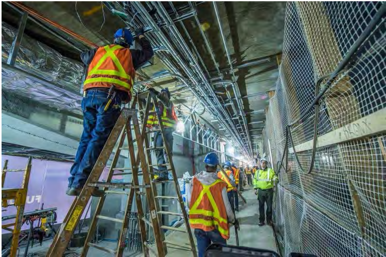
Installation of conduit at the Cortlandt St station.
